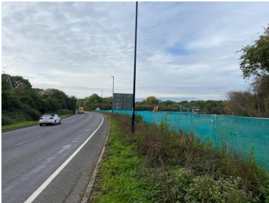
Photograph 4: View looking southwest along Jane Murray Way.
