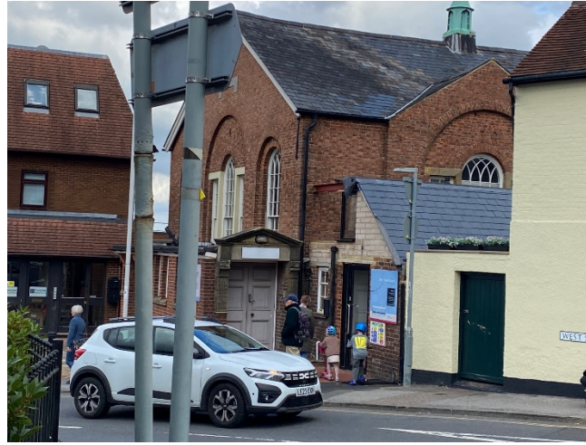
Current View from Ship Street
