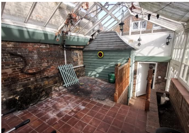
Figure 6 – Existing extension internal
