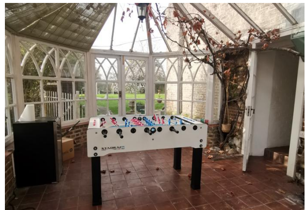
Figure 7 - Existing extension internal
