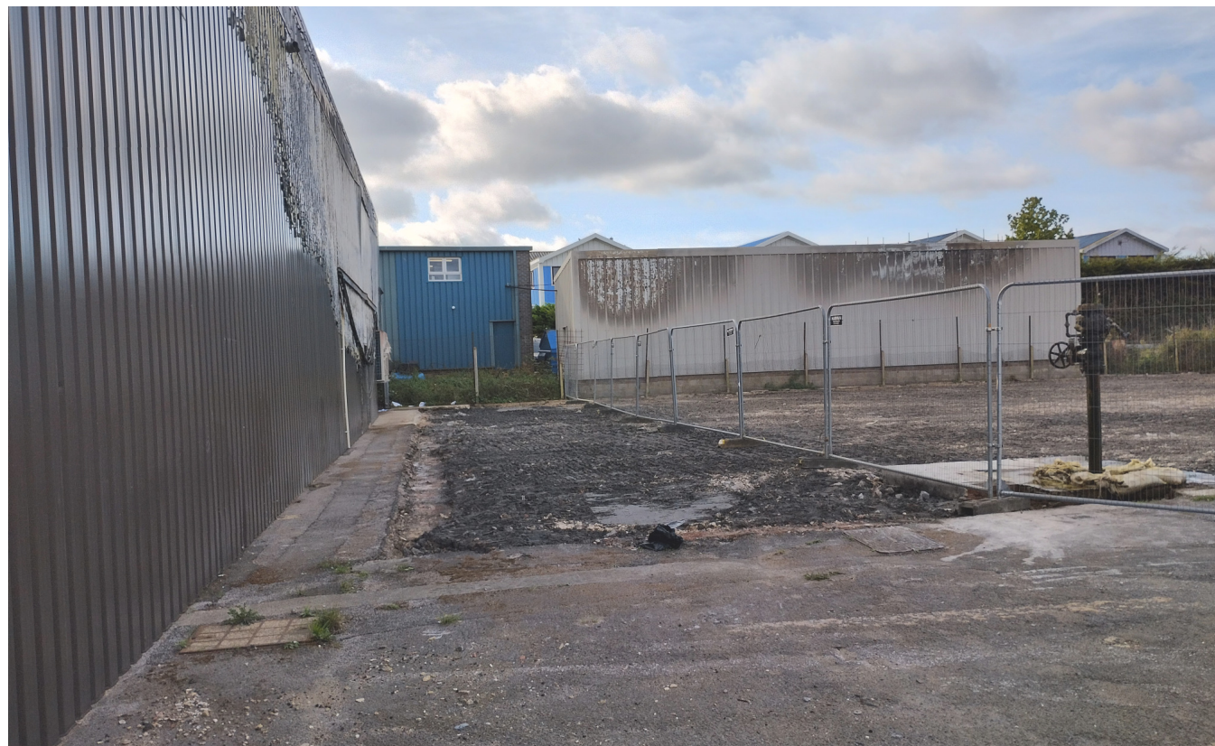
Post fire - View including adjacent building
