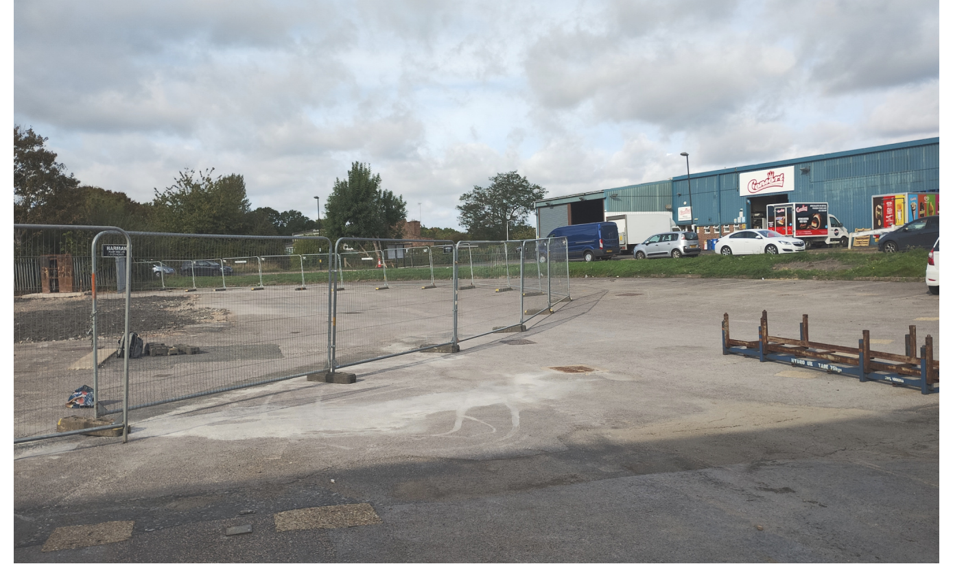
Post fire - View from grass verge
