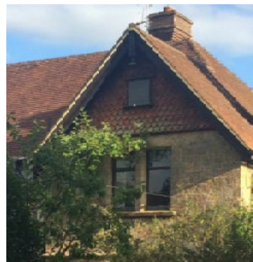
Fig.11 Hung tiling to gables
