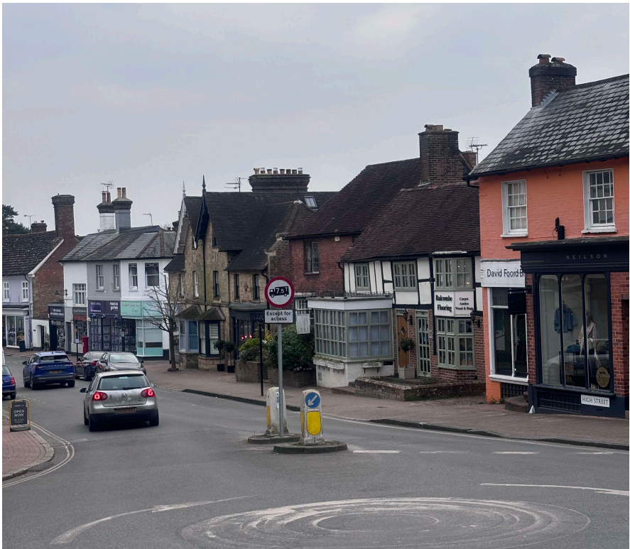
Photograph 6. distance view of main roof slope (north) from upper High Street
