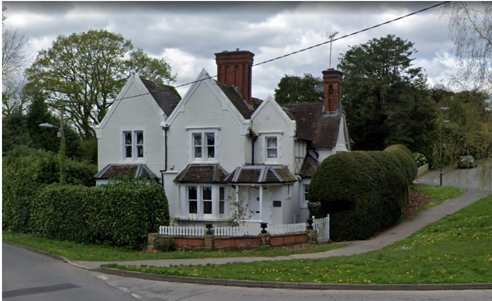
Figure 1 - View of 'Finches Corner' from Hickmans Lane. (Google Maps).
