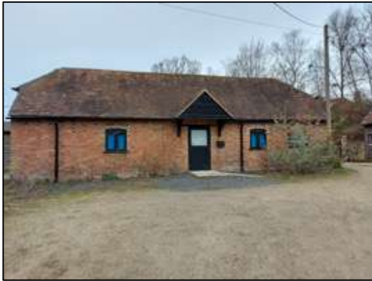
Photograph 1: Eastern elevation of building B1 (Photograph taken by Thomas Knight 17 th March 2021).
