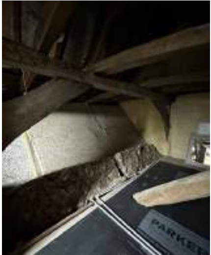
Attic, view of the vaulted ceiling
