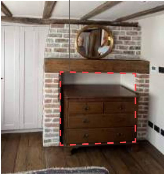
First floor bedroom re-faced chimney breast
