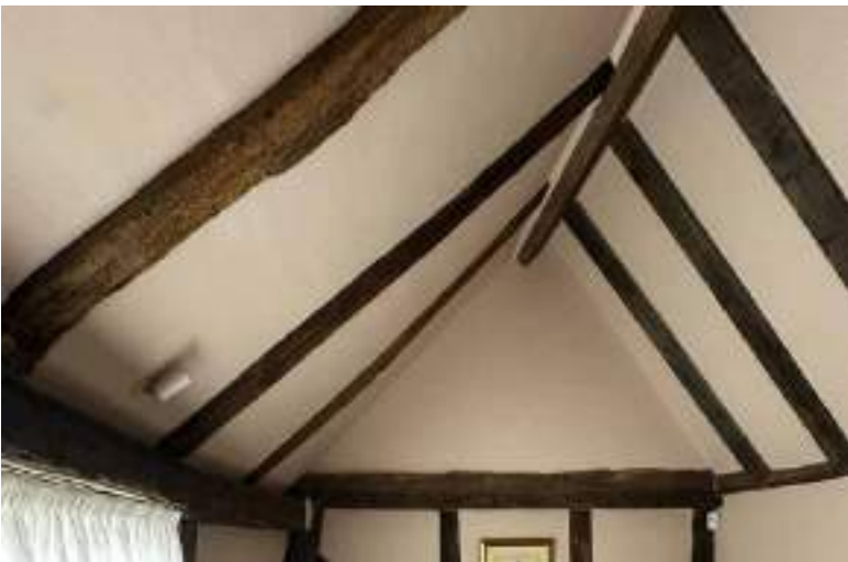
Vaulted Ceiling in SE Bedroom
