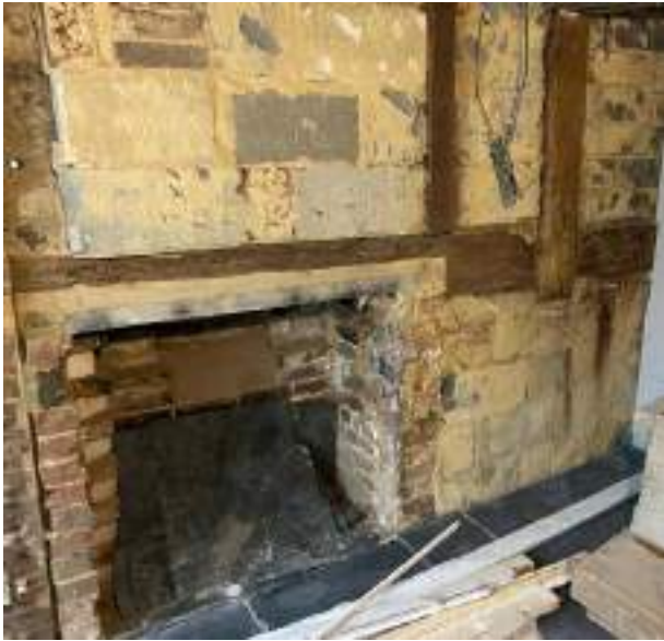
Ground floor living chimney breast under construction, prior to re-facing. Non-original blockwork wall infill exposed.
