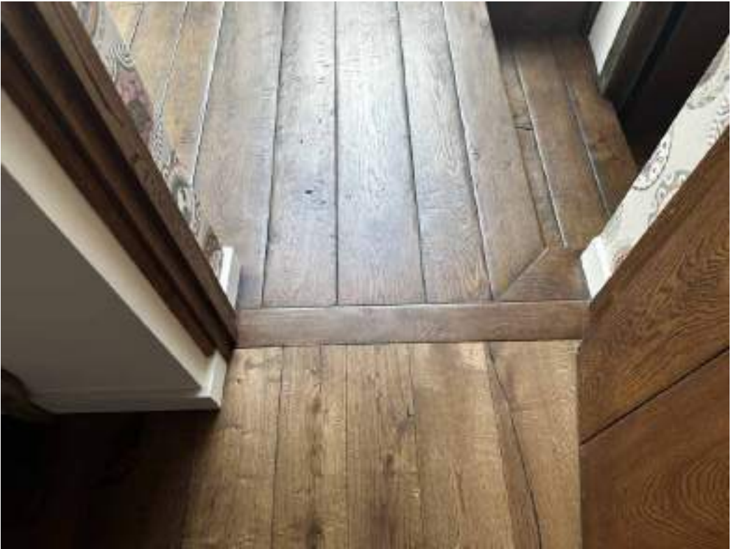
As-built oak flooring
