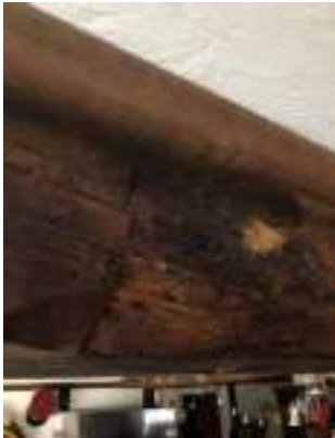
Photographs of oiled oak joist prior to restoration
