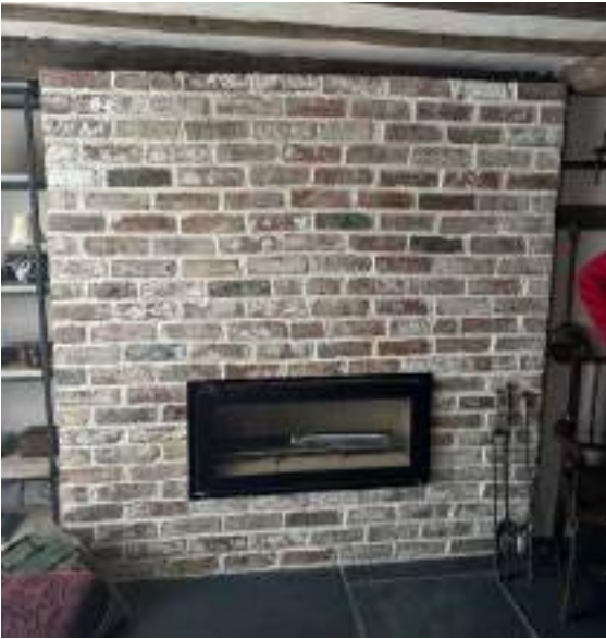
Ground floor living room re-faced chimney breast
