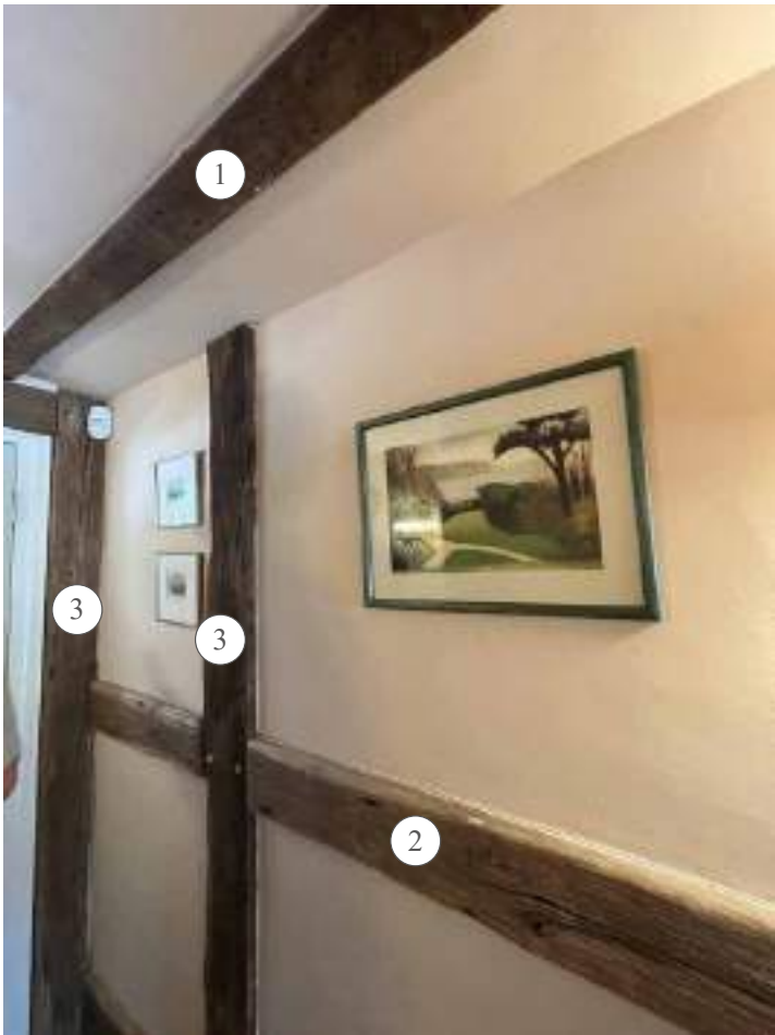
Recent photograph of the hallway wall
