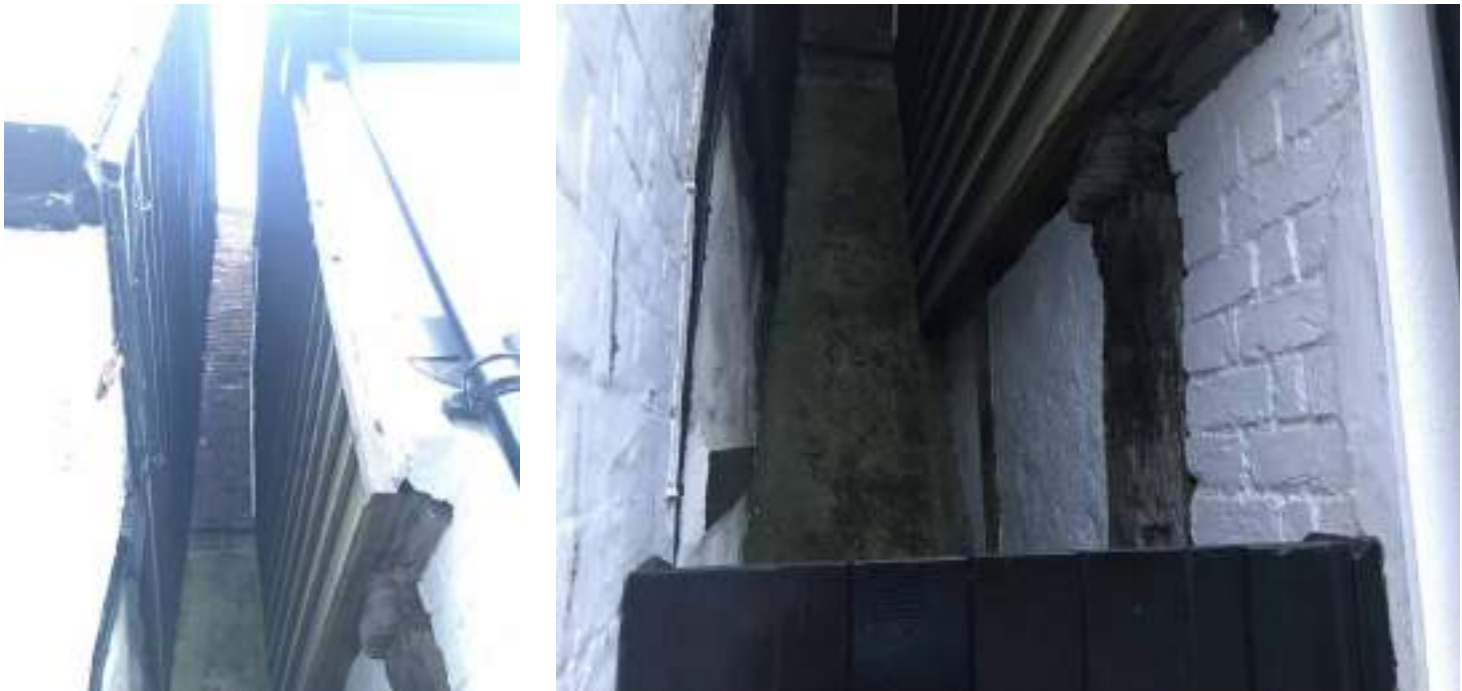
Recent photographs of timber weatherboarding
