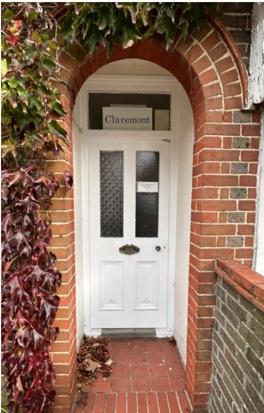
Existing door. Four panel door with glazed upper panels, solid lower panels & transom window.
