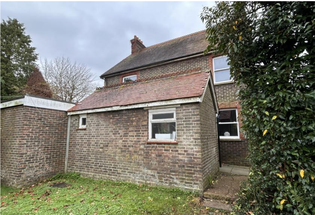
View of the rear of Claremont, with external Store outbuilding in the foreground and cold store building adjacent on the left.
