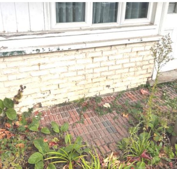
Shop front original brick paving
