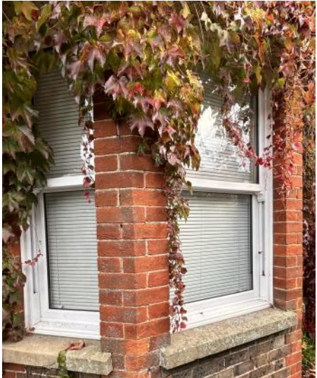
Existing front bay windows in heritage style uPVC—to be retained & matched.
