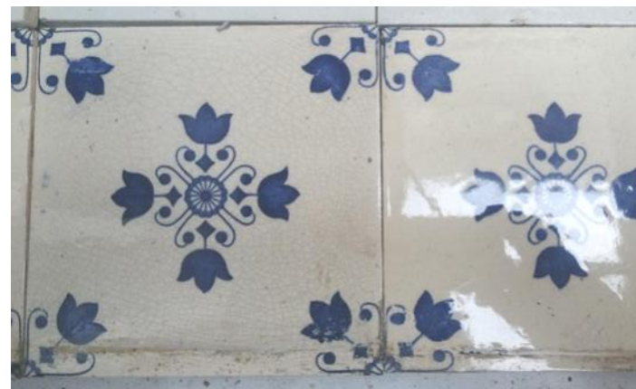
Original tiles to be reinstated
