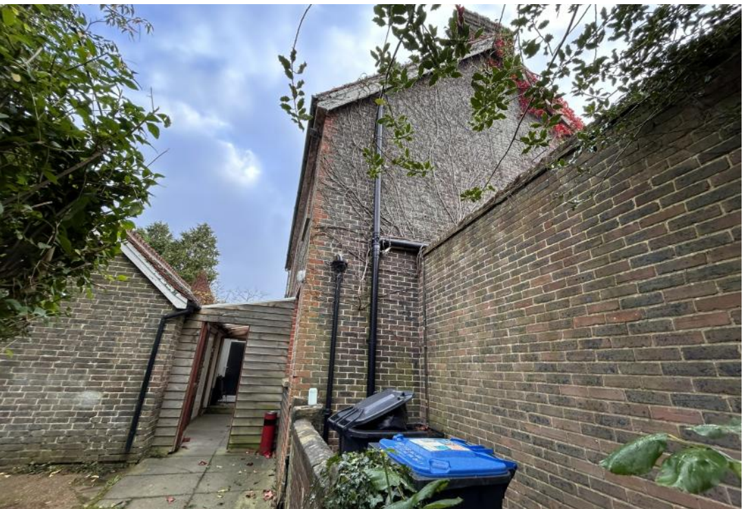
View of the rear of Claremont from the back of the West extension looking towards the Outbuilding/ rear entrance.
