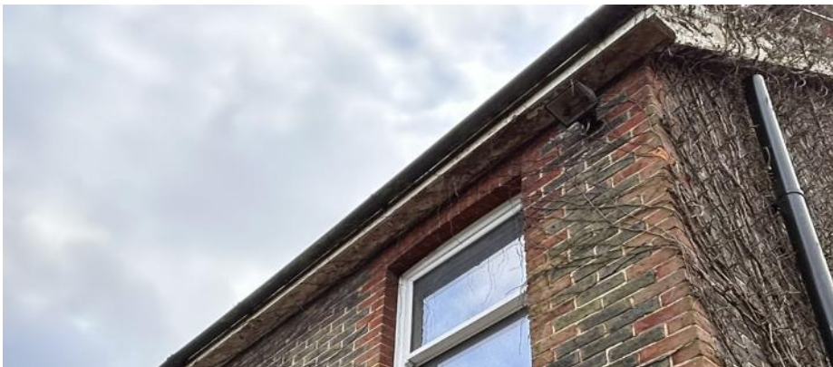
Existing & new roof eaves with closed soffit in box type painted wood. No visible eaves ventilation fixings.
