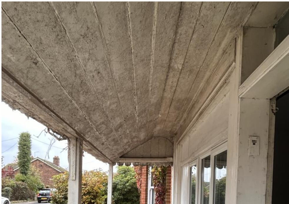
Shop canopy timber panelled soffit
