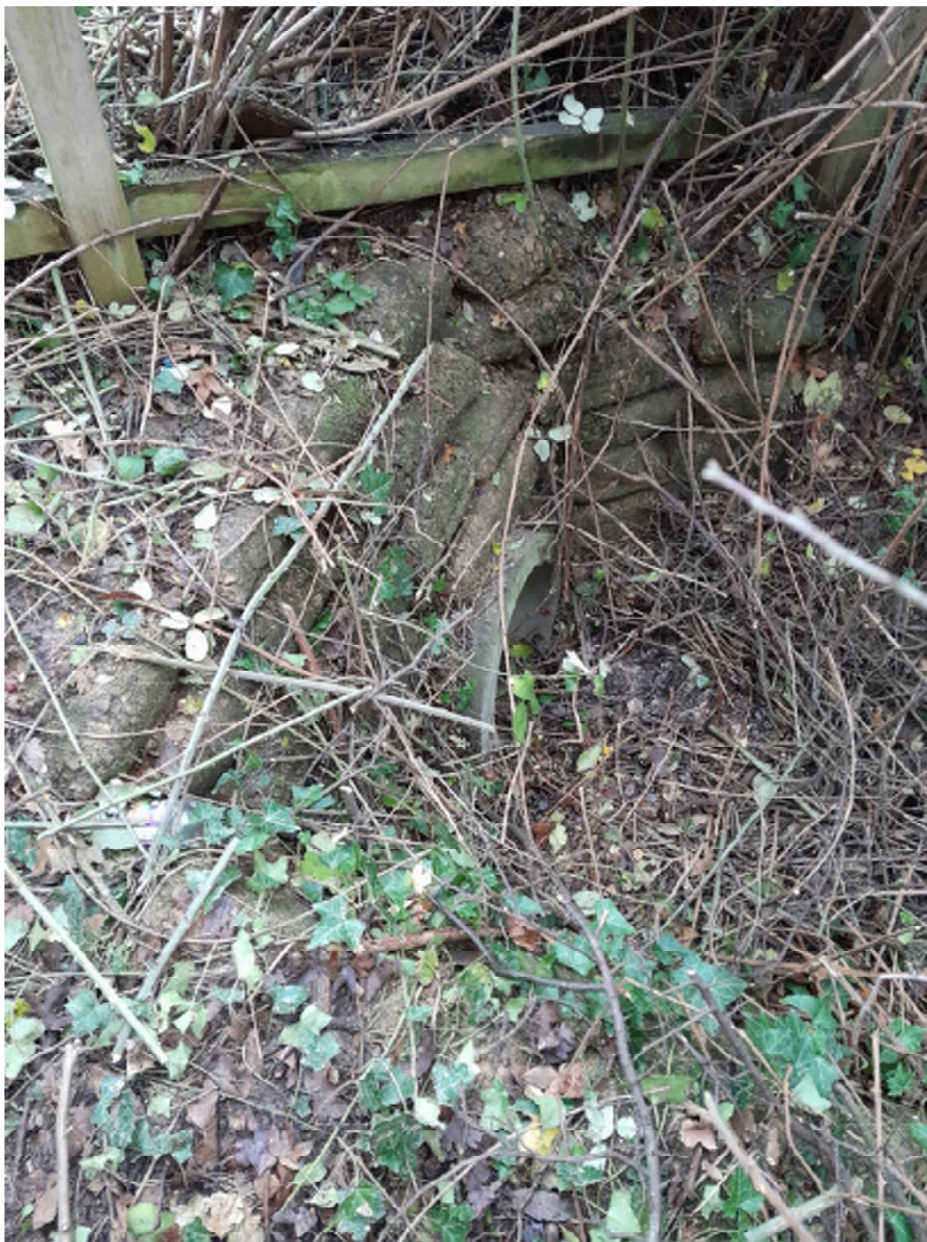
A2300 Culvert entrance – November 2022
