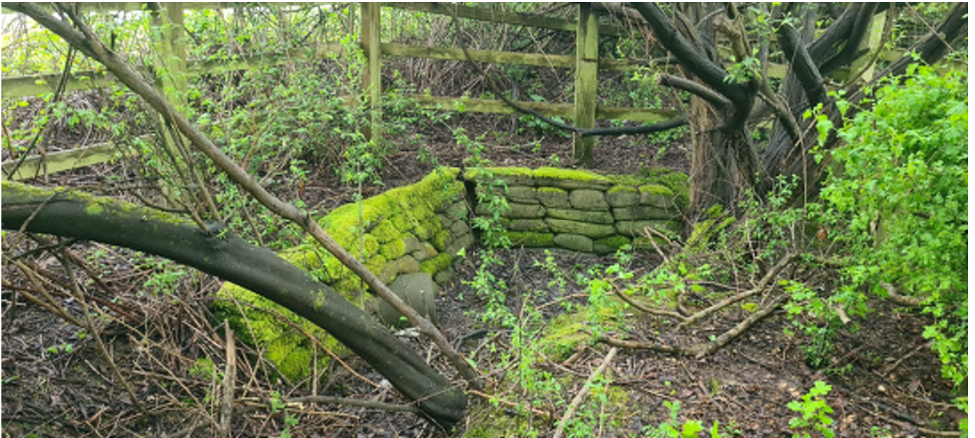
A273 Culvert Outfall to ditch on west side of A273 – May 2024
