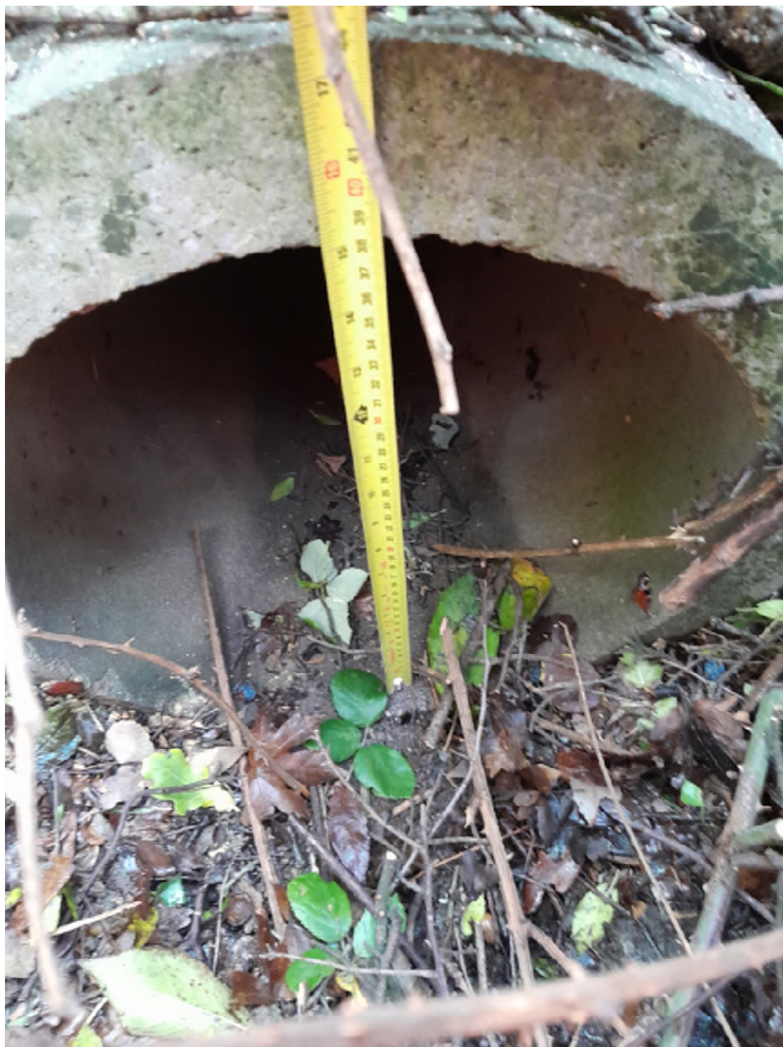
A2300 Culvert entrance – November 2022
