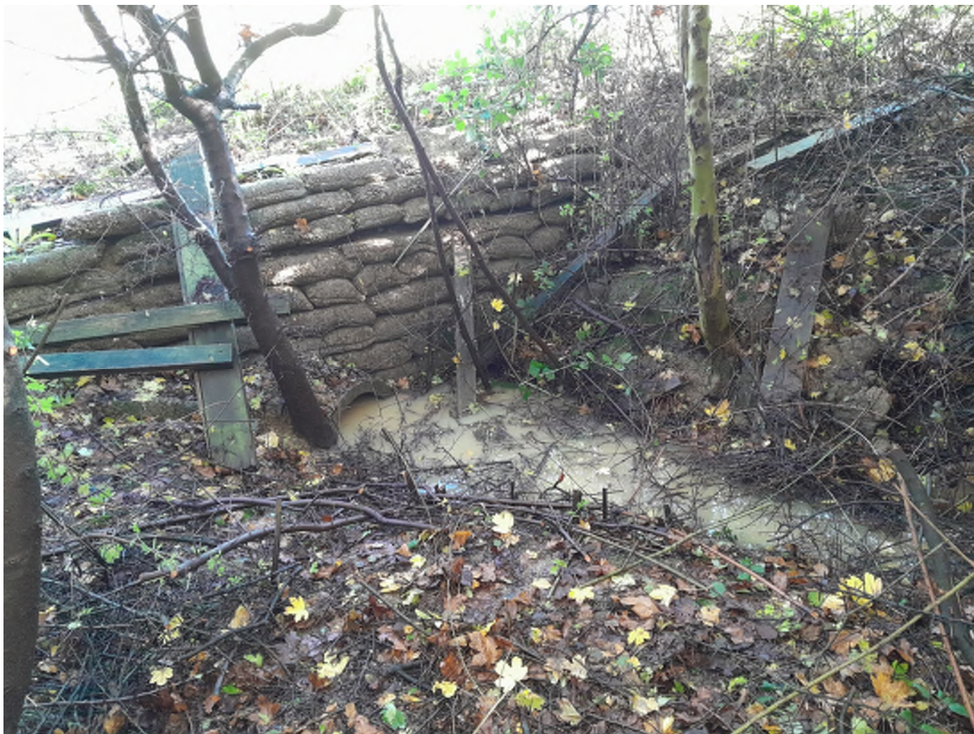
A2300 Culvert outfall – November 2022
