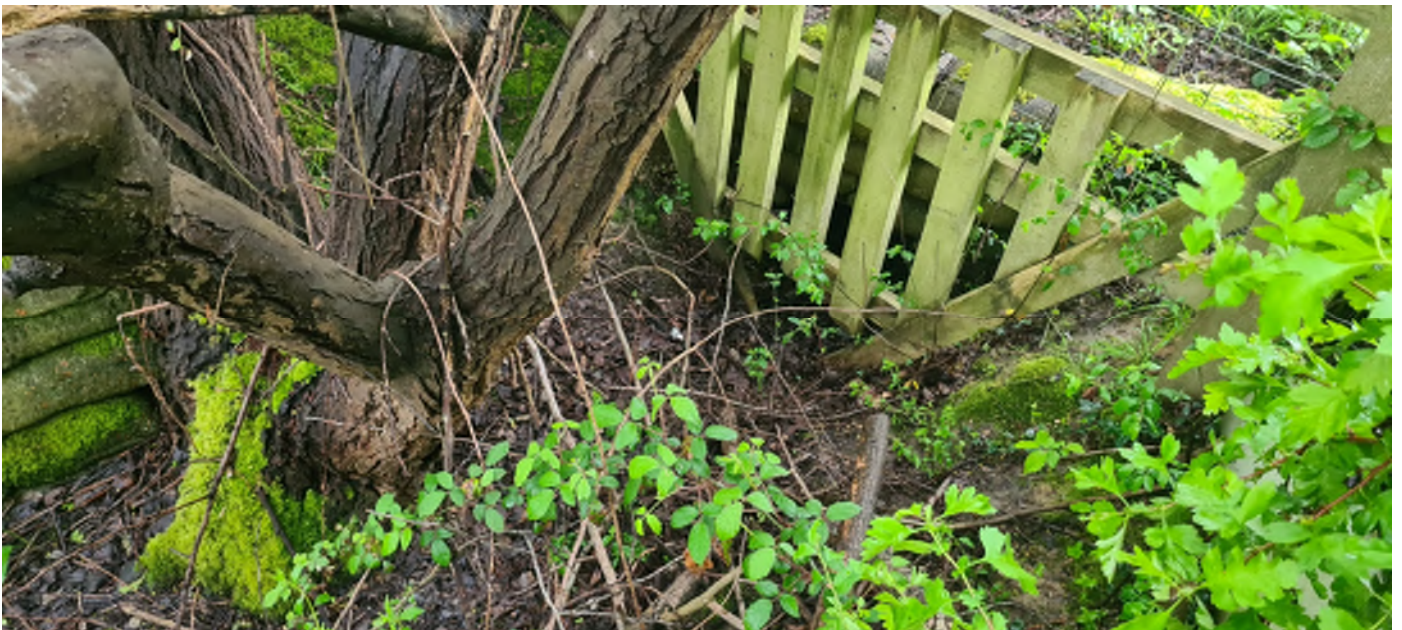
Ditch on west side of A273, at entrance of field culvert (ditch passes under timber fence into culvert entrance. Concrete bag work headwall just visible through fence)
