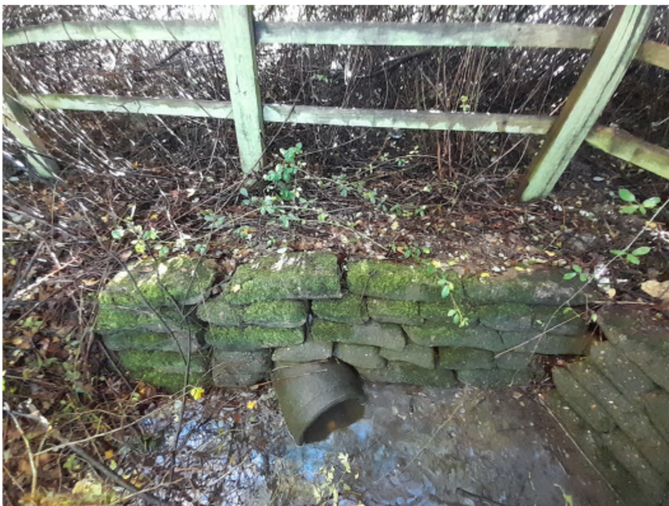
A273 Culvert Outfall to ditch on west side of A273 – November 2022
