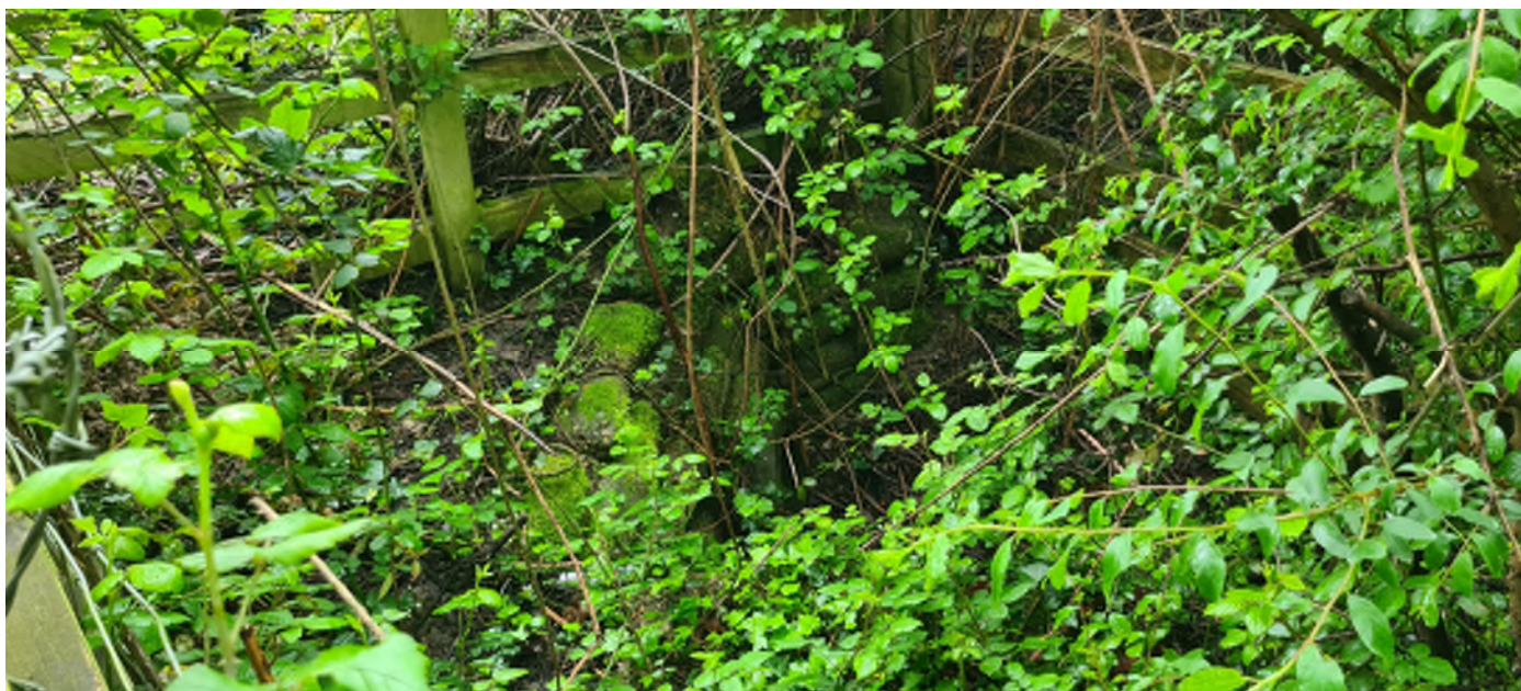
A2300 Culvert entrance and headwall – May 2024
