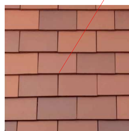
Roof cladding match
