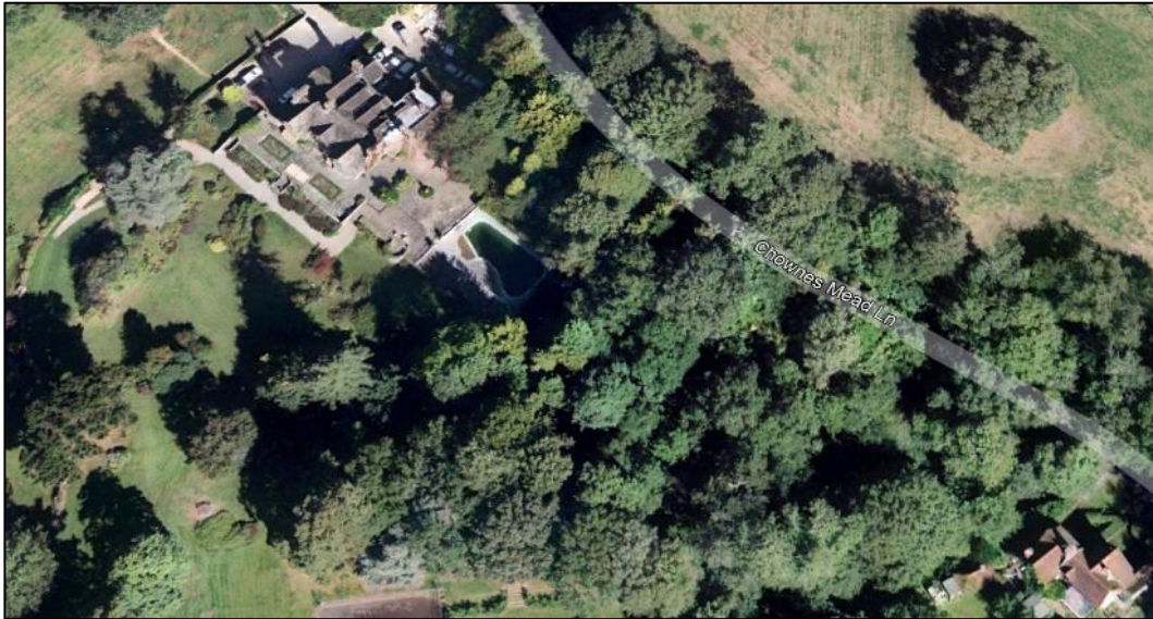
Figure 2. Google Earth, aerial image from 31/08/2012
