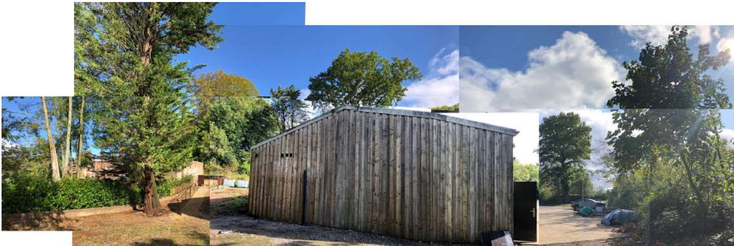
E02 - Looking East towards timber clad barn
