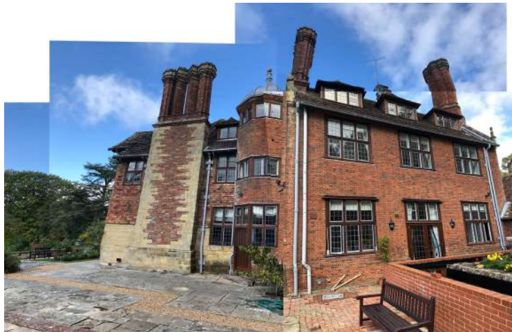
B03 - Looking North West towards Chownes Mead
