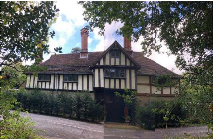
A01 - Looking West towards the Coach House from Chownes Mead Lane
