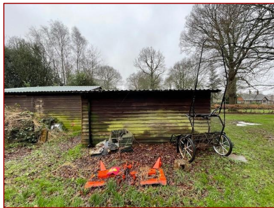
Photo 1 – North Elevation of Straw Barn
