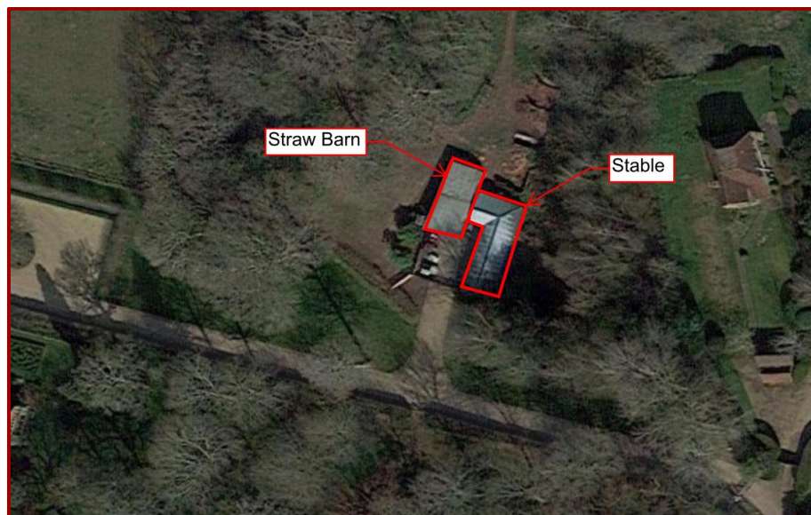
Fig 4.1 – Aerial Photograph of site
