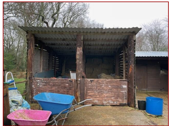
Photo 3 – South Elevation of Straw Barn
