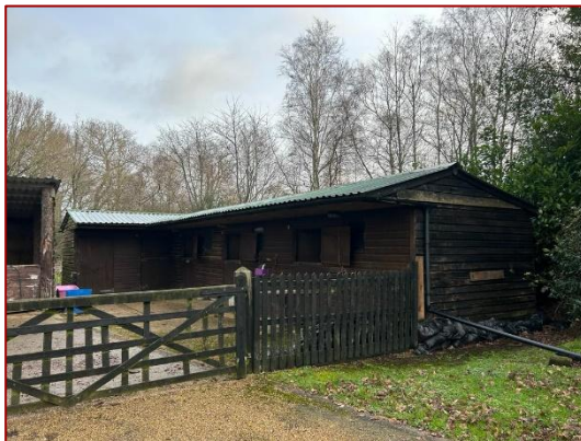
Photo 5 – South and West Elevation - Stable
