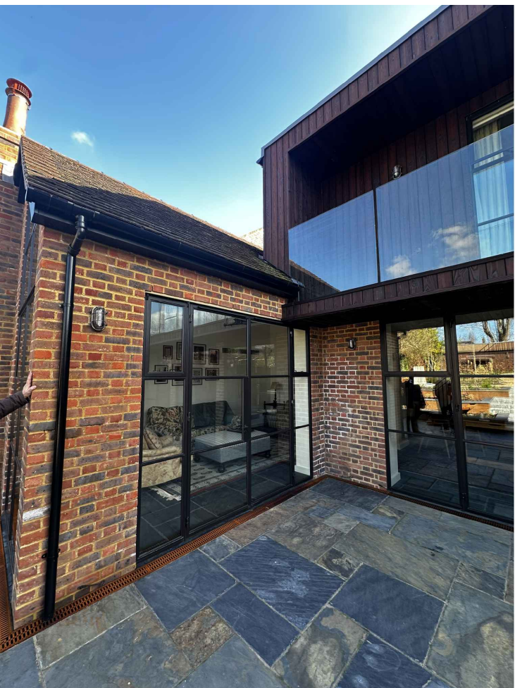
Bake house, South elevation
