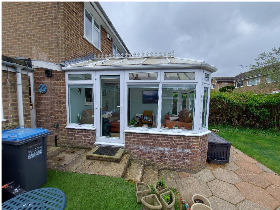
North East Elevation of existing conservatory
