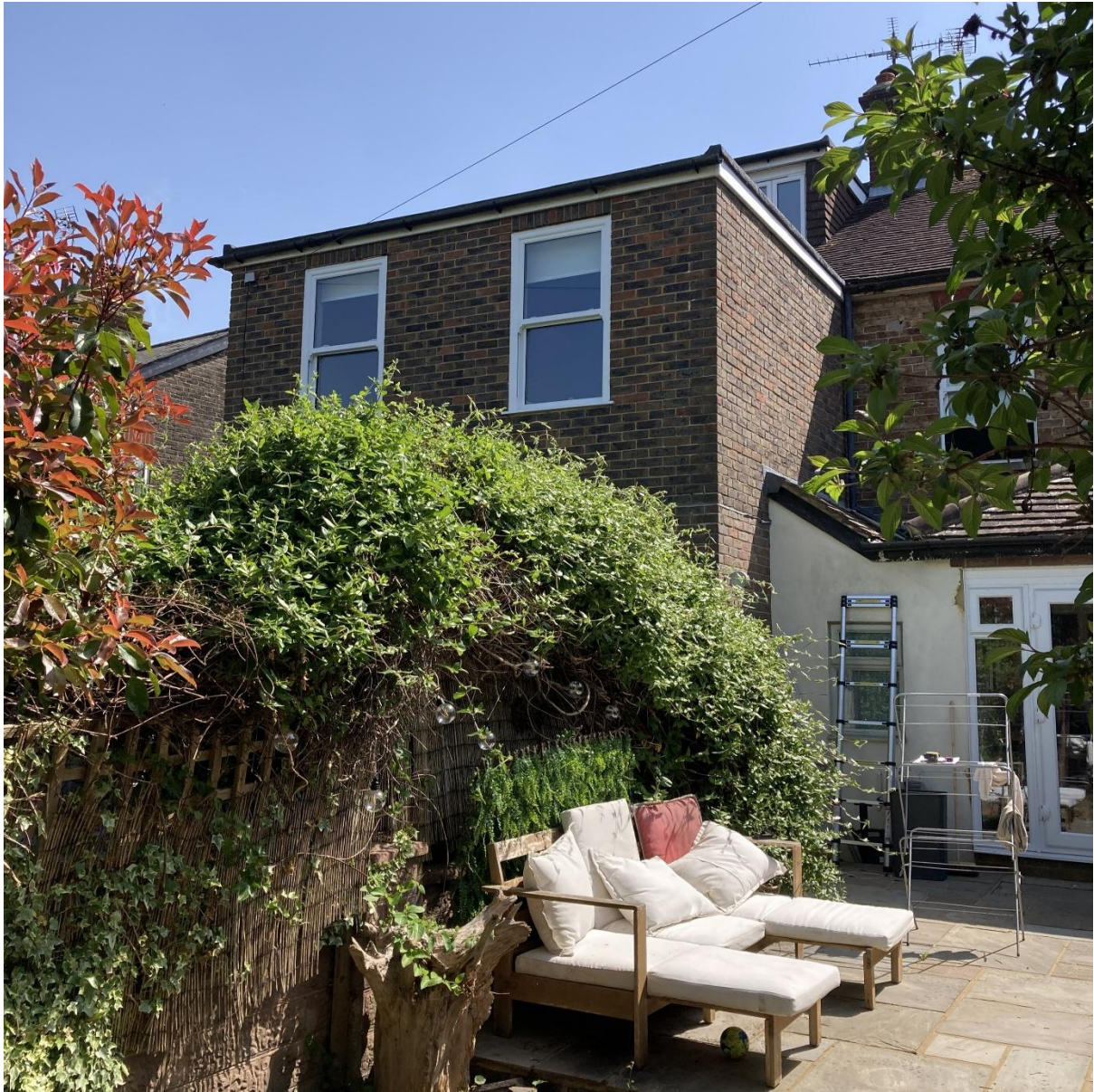
Image 03: 56 Western Road, Hurstpierpoint – Rear Extension & Rear Dormer
