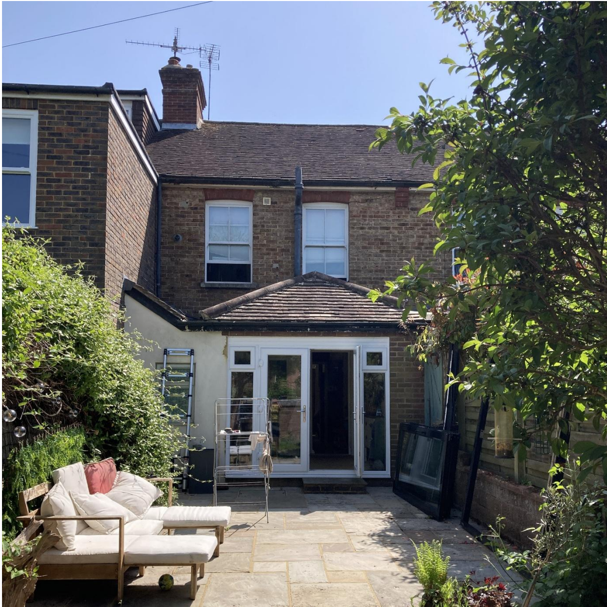
Image 02: 54 Western Road, Hurstpierpoint – Rear Elevation
