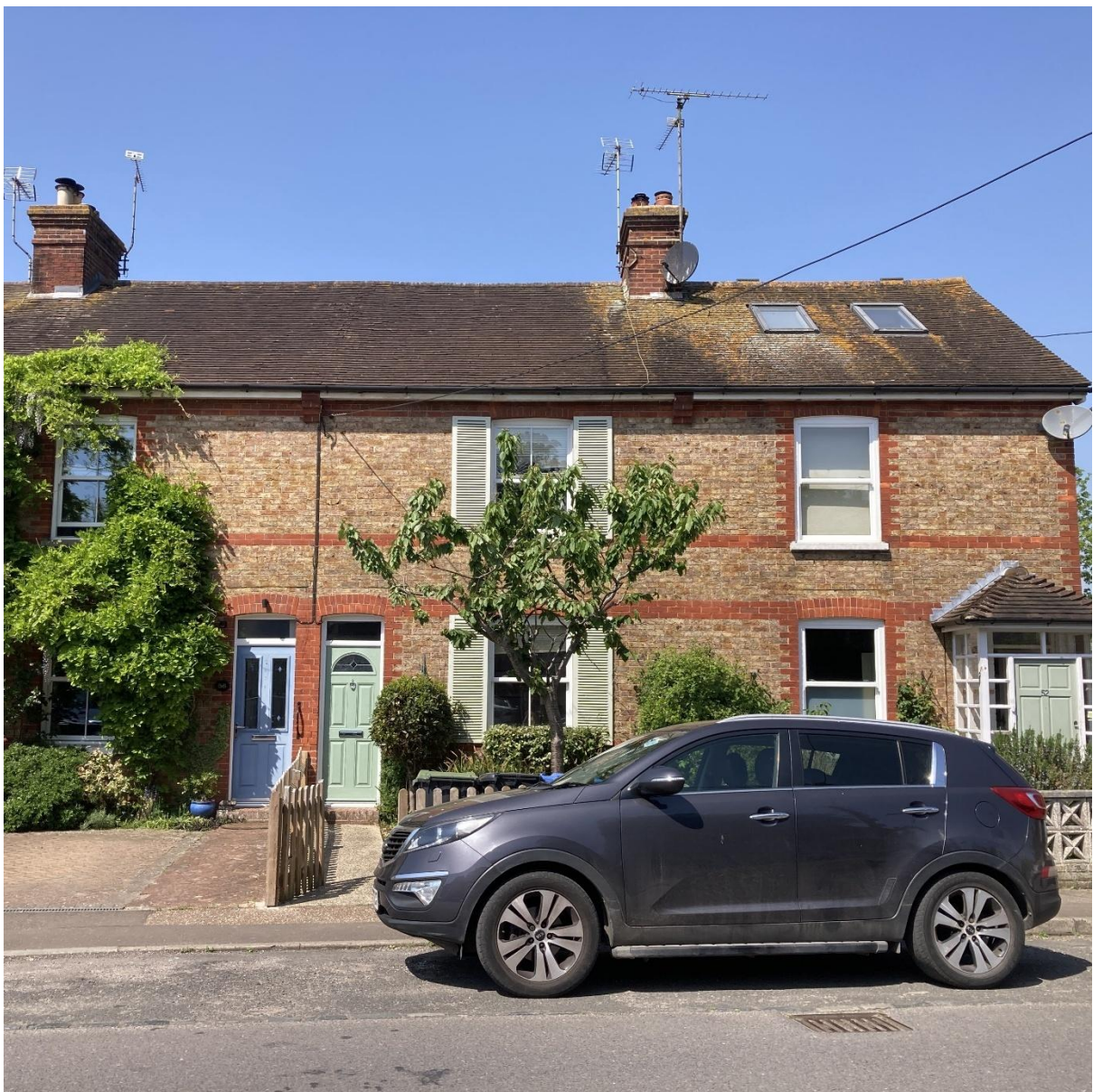
Image 01: 54 Western Road, Hurstpierpoint – Front Elevation
