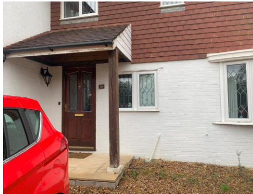
View of existing open sided porch
