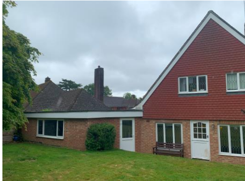
View towards existing garage
