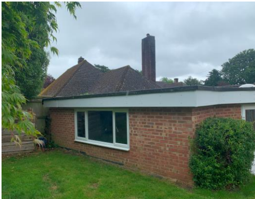
View of existing garage facing rear garden
