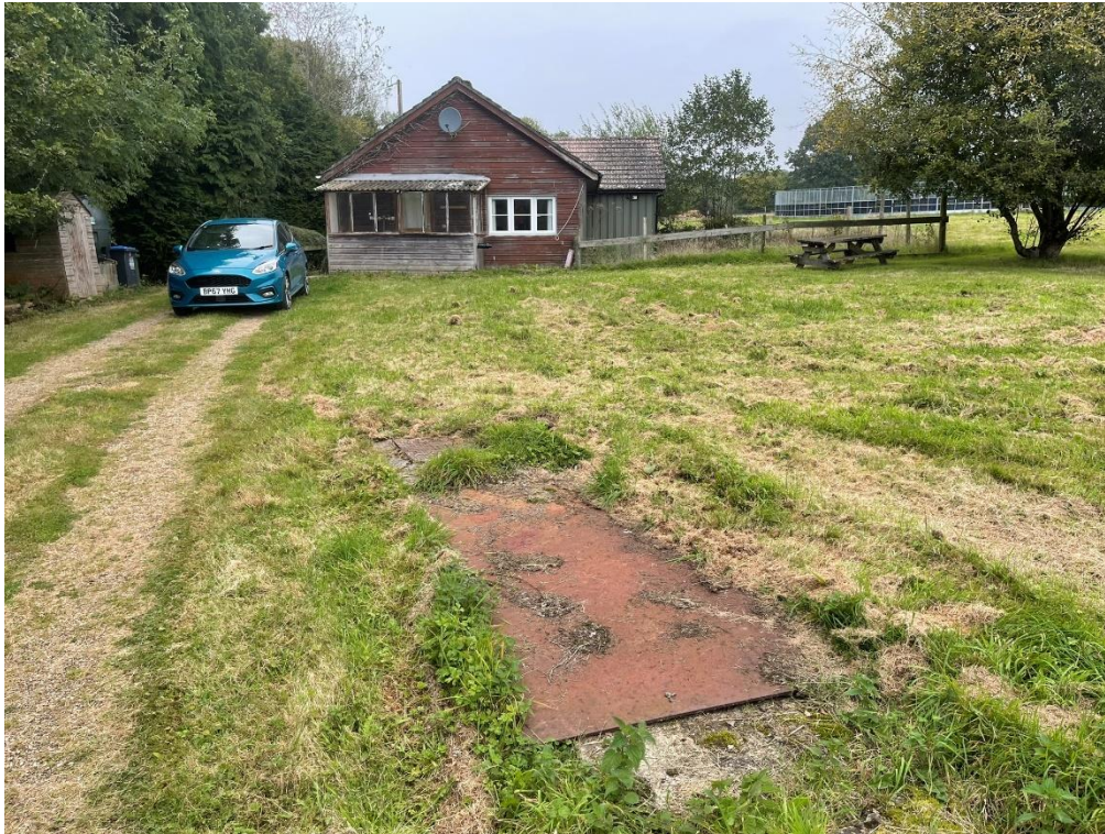
Image 01 – Showing the existing Dwelling and the septic tank / foul treatment plant
