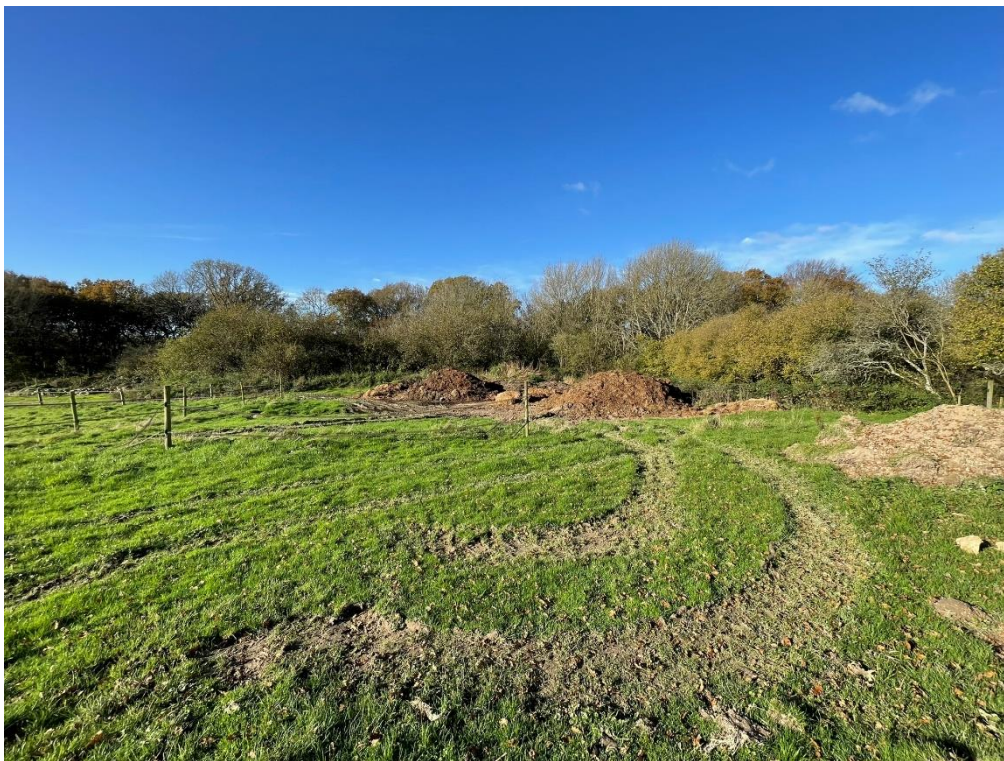
Image 02 –A view of the proposed dwelling location, looking East with the groundworks to the garage already progressed
