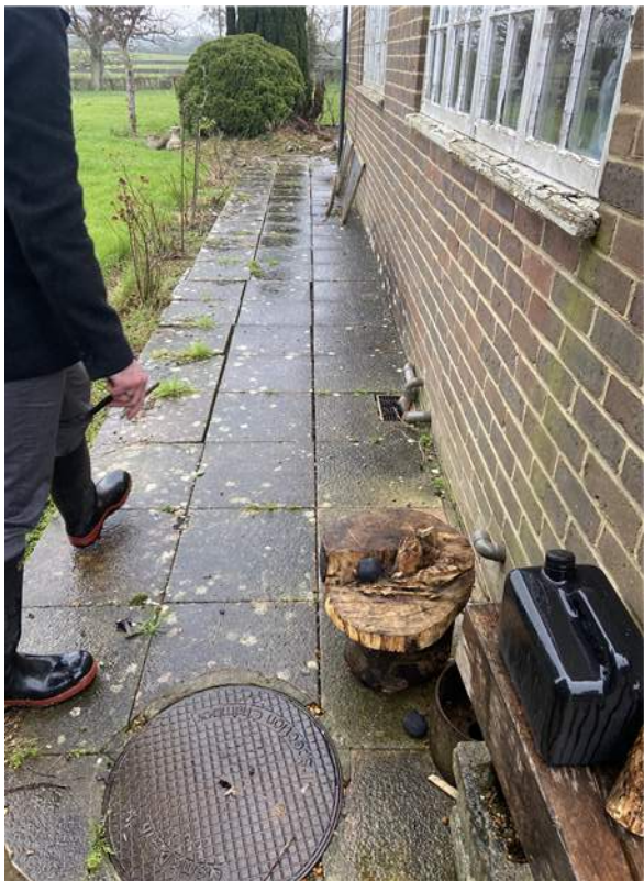
G02 / MH03 G02 in background - gully pot for kitchen greywater MH03 in foreground
