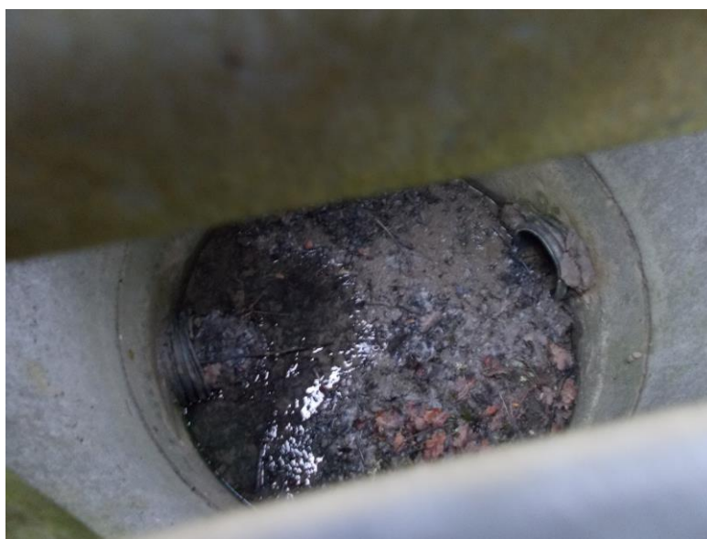
Internal view of the 1 st chamber
