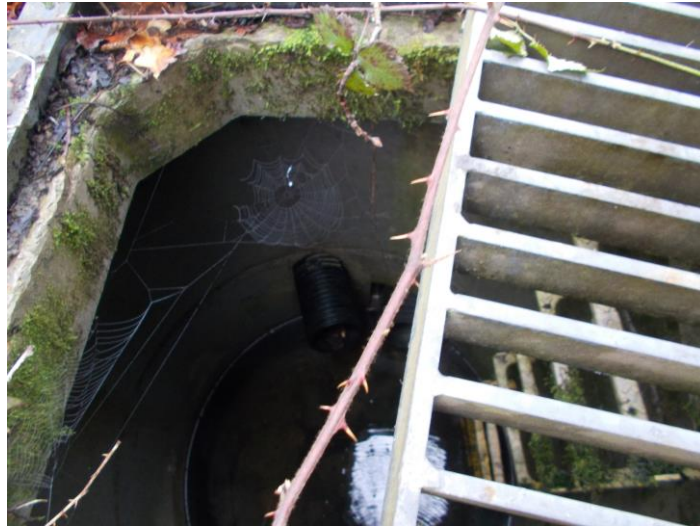
Internal view of the 4 th chamber, with drainage ditch from the Taylor Wimpey site (from the east) joining the watercourse (already draining from the south, past the Site A). The watercourse flows northwest under in embankment via this chamber.
