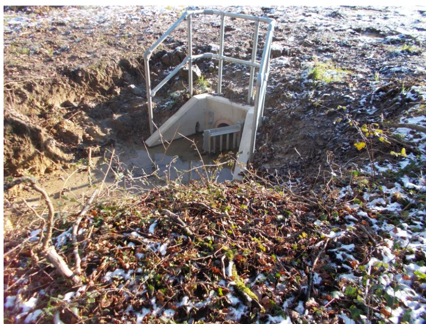
Ditch at the northeastern boundary of the site used by Taylor Wimpey for Surface water SuDS drainage.
