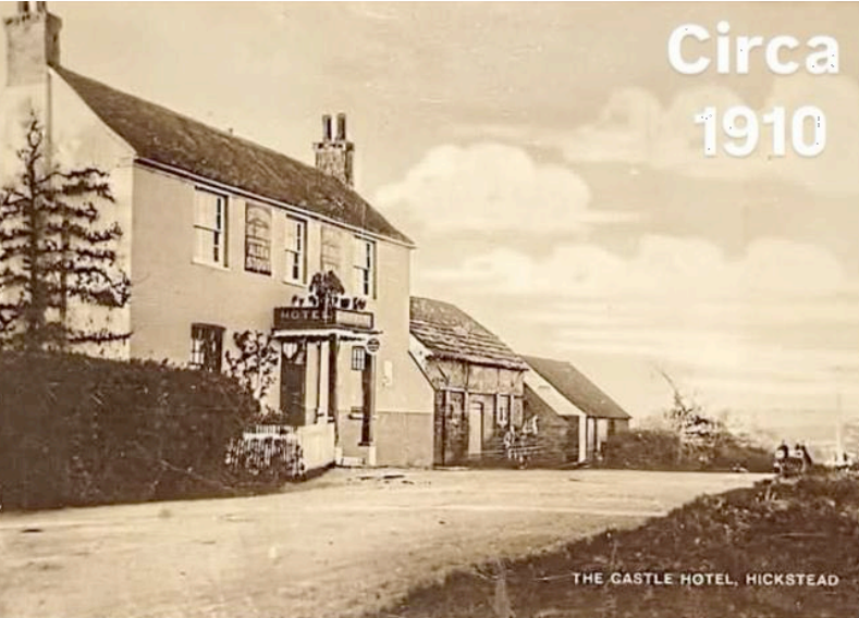
HISTORIC PHOTOGRAPH, c.1910 SHOWING ENTRANCE CANOPY
