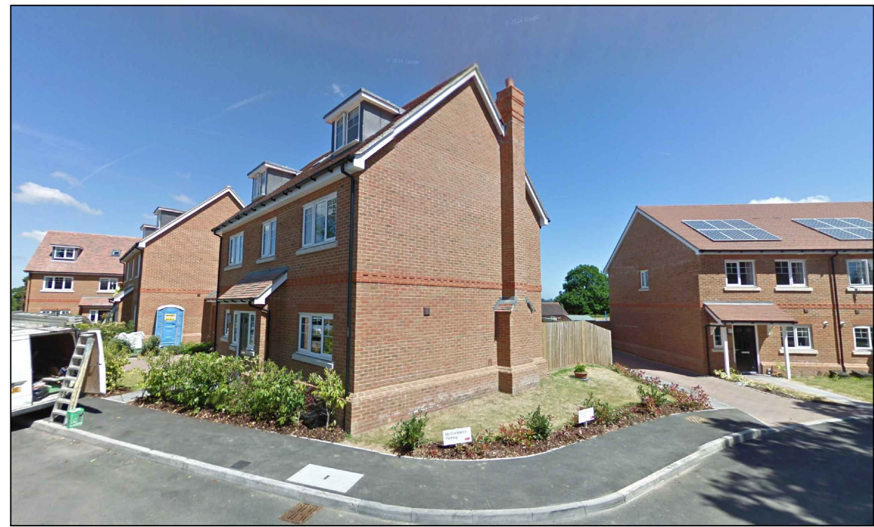
Original Site Photos - 5 Beacon Rise
