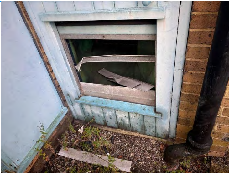
Ventilation system associated with the tank
