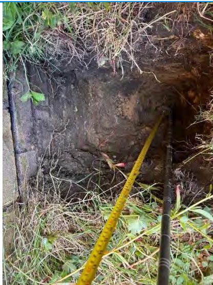
TP02 showing existing foundations
