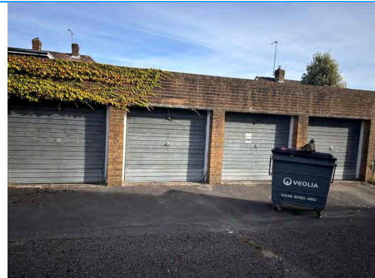
Garages towards the north of the site
