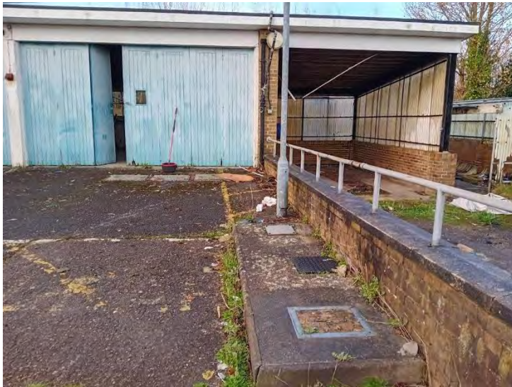
Possible tank covers and a pump island on the northwest of the site.
