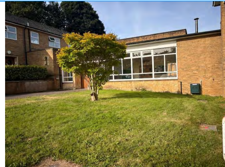
Western view towards the front of former police station building
