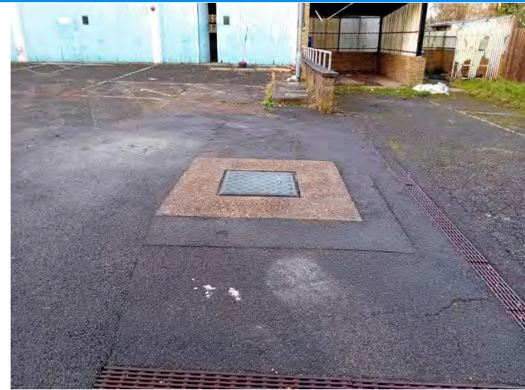
Suspected interceptor on the north side of the courtyard.
