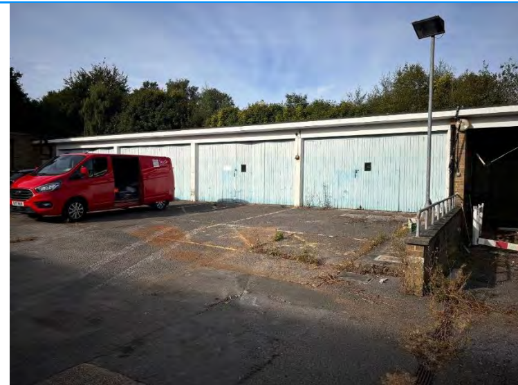
South-western view of existing buildings likely formerly used for vehicle storage
