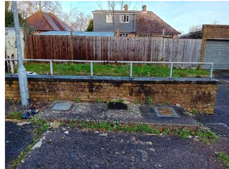
Suspected pump island.
