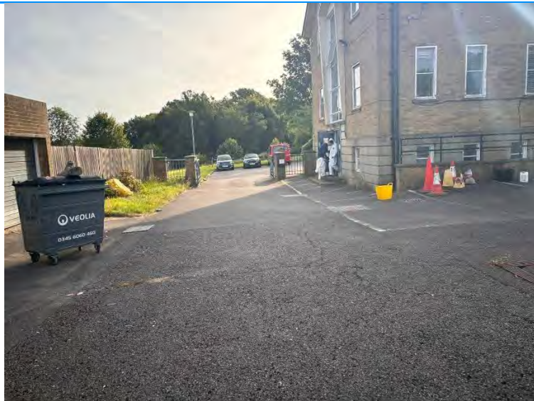
View towards the east showing the former police station and asbestos removal
