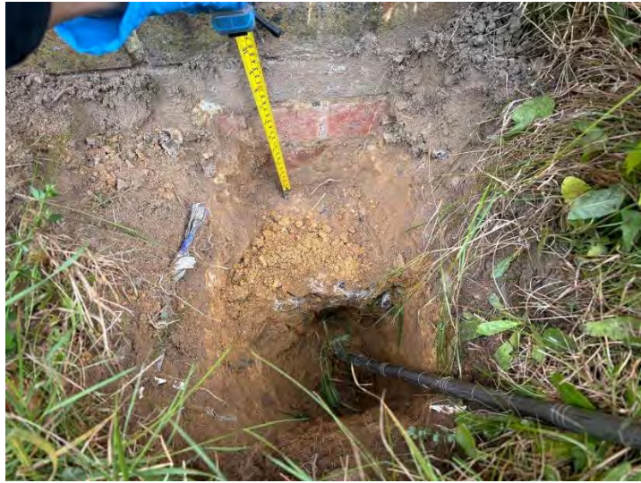
TP01 showing existing stepped building foundations
