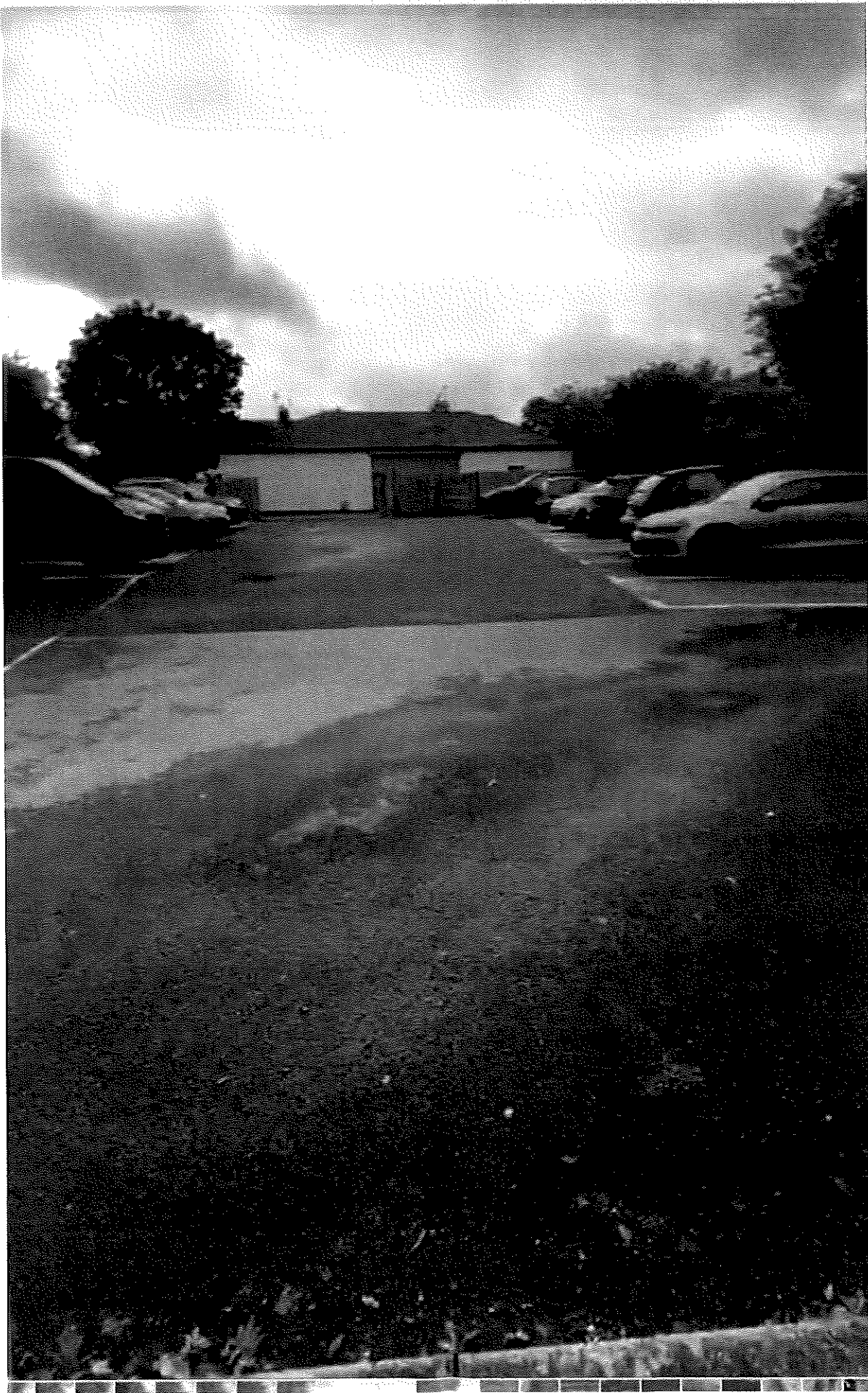
Photo To Show Access To Site
