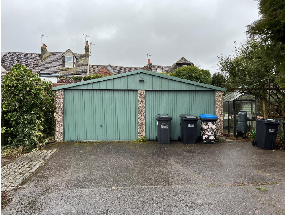
Photo Above: The Existing Double Garage to be Replaced
