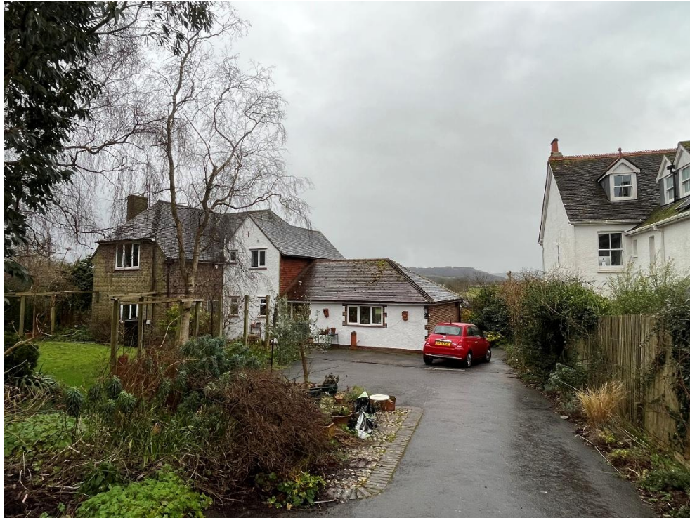
Photo Above: Front Elevation of Culvers
