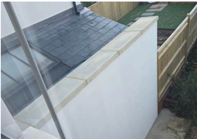
Fig. 10: Photograph of neighbouring extension (No.142) with matching buff coping stone.
