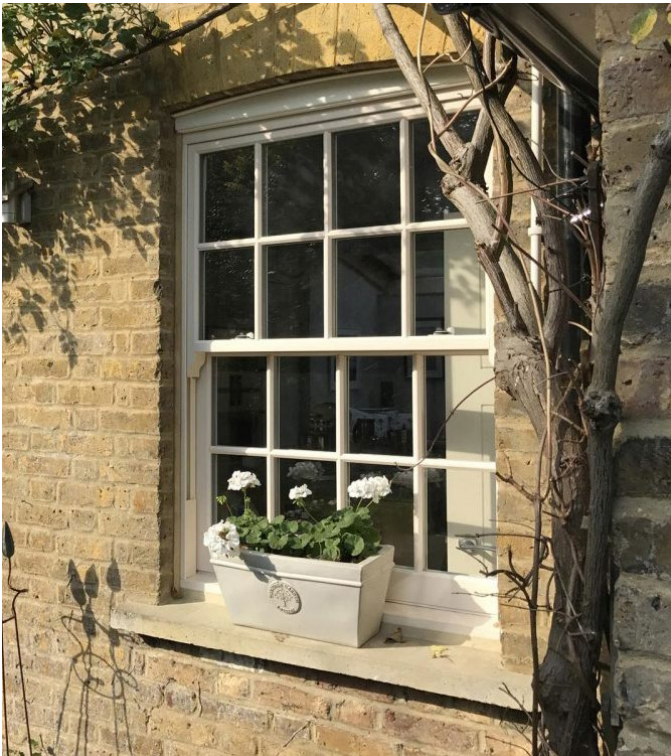
Fig. 20: Example of identical product installed from Roseview Windows (supplier).
