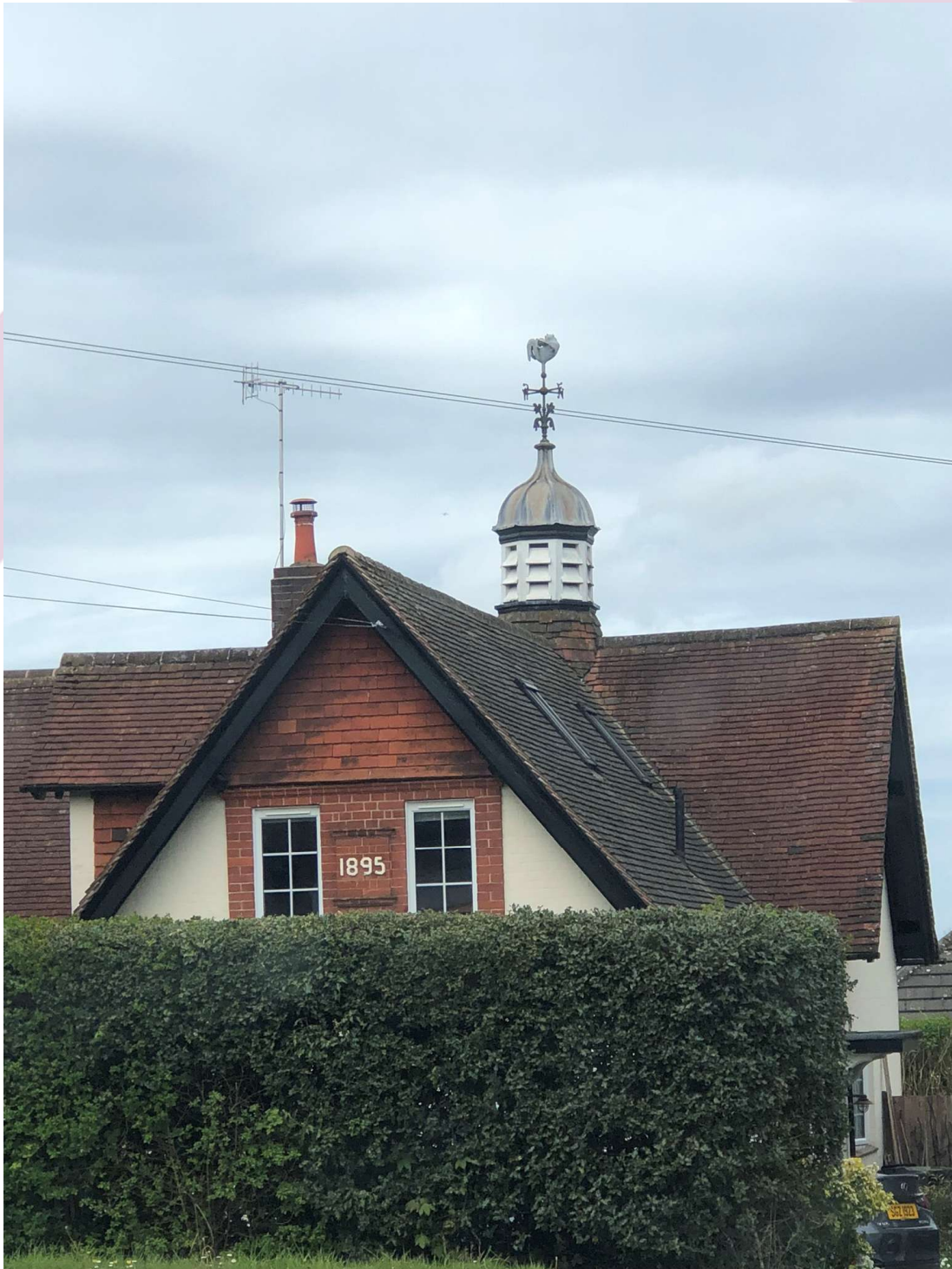
Figure 5 Building marked 1895 with a cupola and tiled roof design reference
