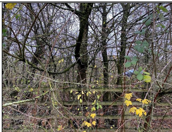
Photograph 10. Timber 'post and rail', fence along the verge of the A23 on the western boundary.
