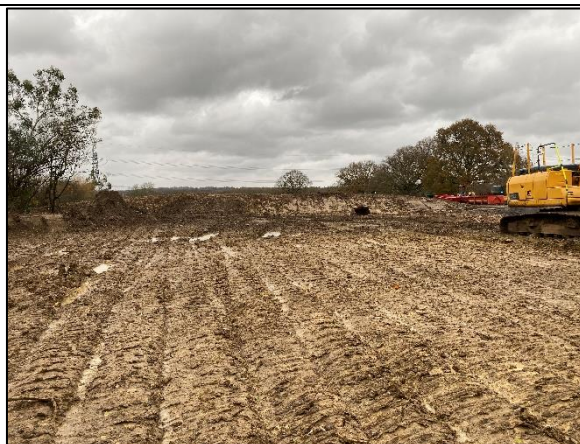
Photograph 14. Recent earthworks adjacent to the entrance.
