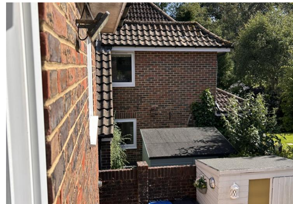
Side View towards No.29 of side-facing windows. The ground floor window is a secondary window to an open plan living space, with additional windows facing the front and rear. The first floor window is a bedroom / study (the additional window to the rear was bricked up as part of the rear extension to the house). As such, great care has been taken in the planning proposal for number 30 to ensure that the light to these windows is not compromised. The extension is located to the North of these windows and thus there is no loss of sunlight.
