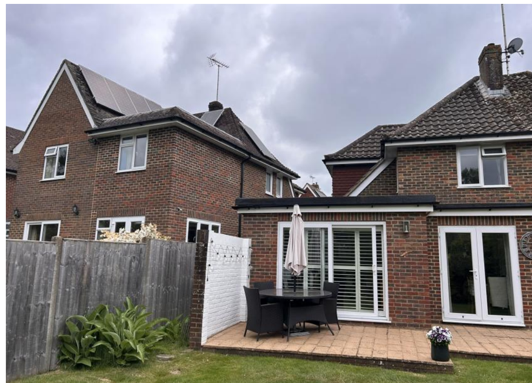
Rear View of No.30 with two storey extension to No 31 visible beyond
