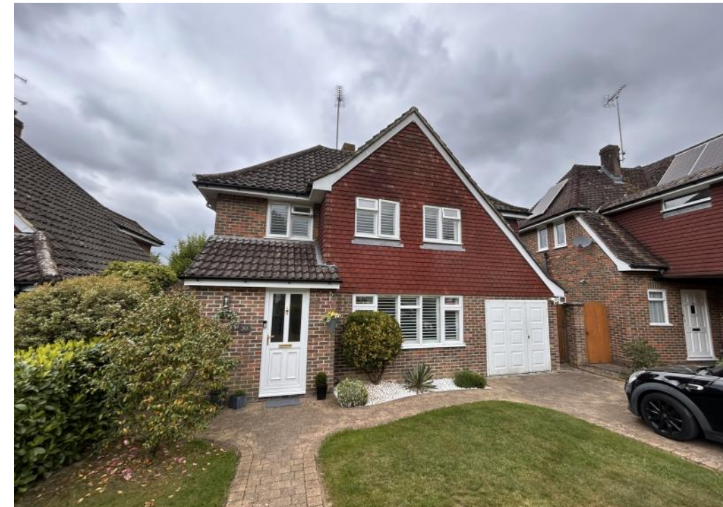
Front street view of 30 Pickers Green
