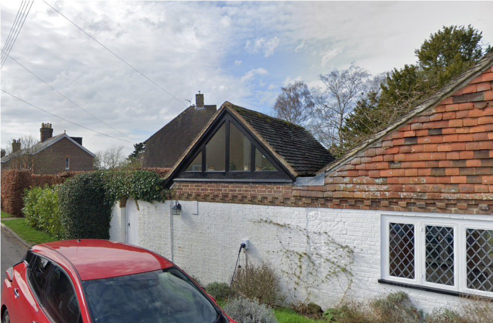
Mulberries roof can be seen from Lewes Rd when positioned next to Rixons. Here it appears behind the pitched gable of the 1990's kitchen extension.
