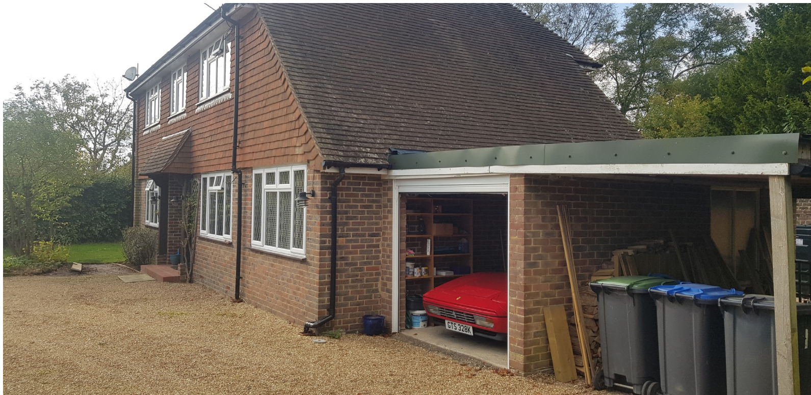
Photo showing existing garage and carport (prior to addition of approved porch - see below)
