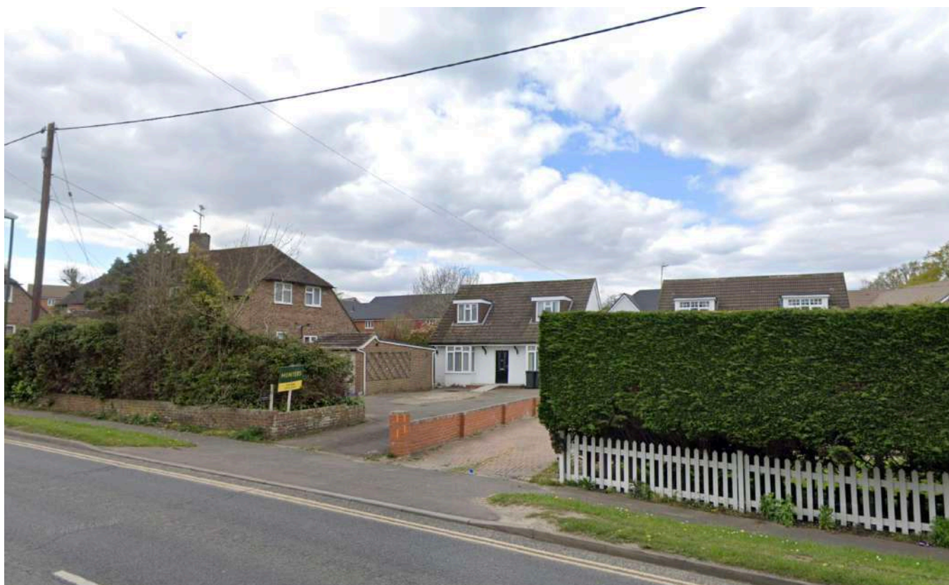
Street view of house and garage from London Road.
