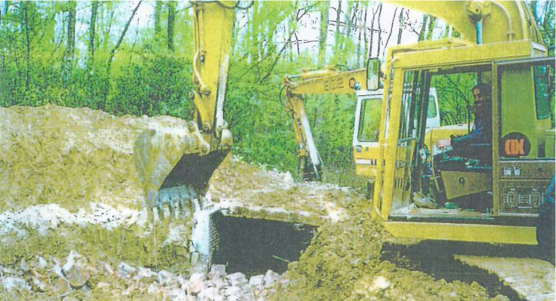
Removal of Entrance to Small tanks
