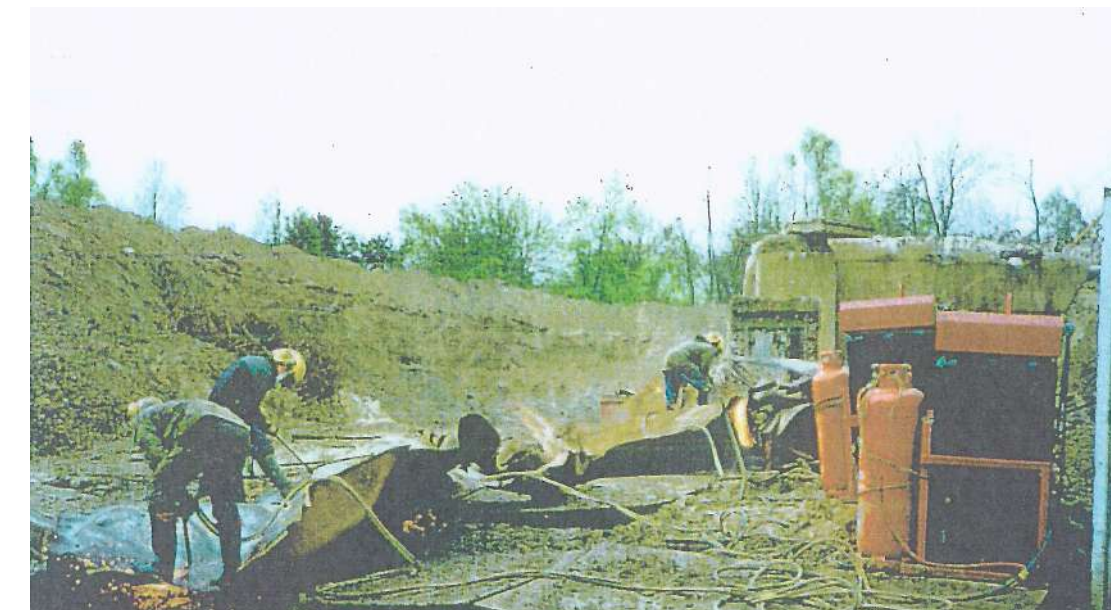
Cutting the steel of the Large Tank
