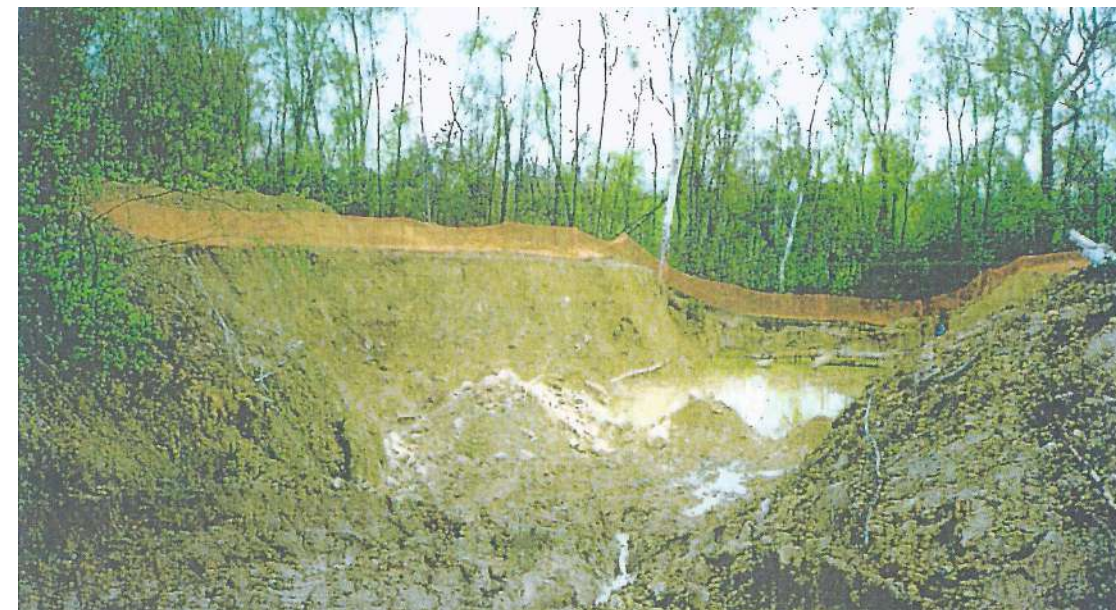
Small Tank after removal of concrete walls - base remains
