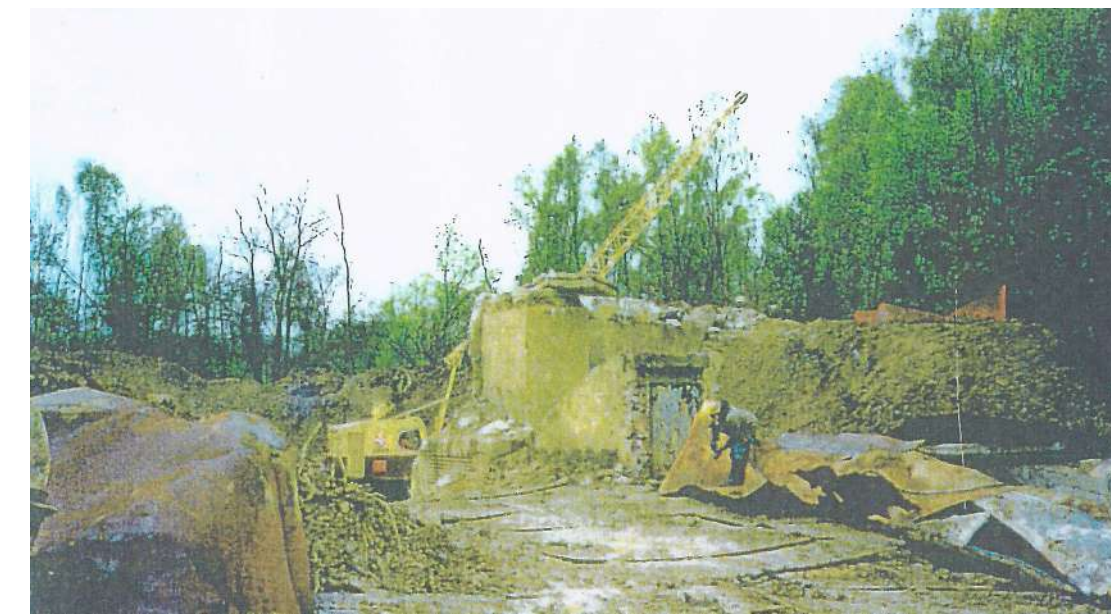
Large Tank with steel removed and concrete being destroyed
