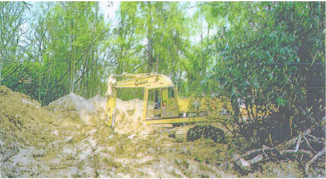
Removal of Small tanks
