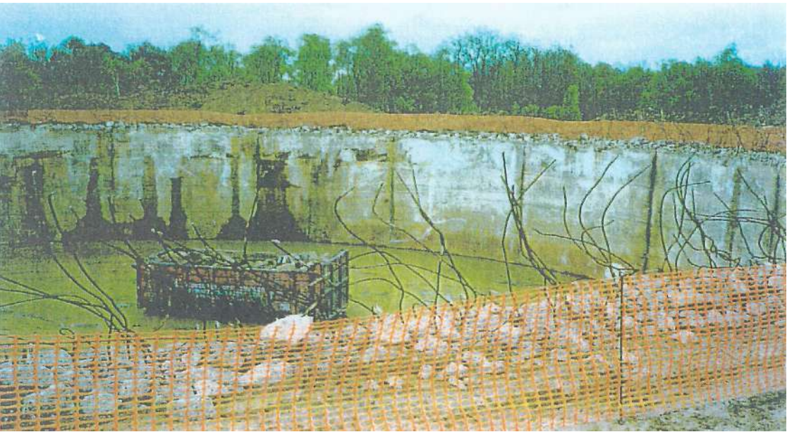
View of Large Tank
