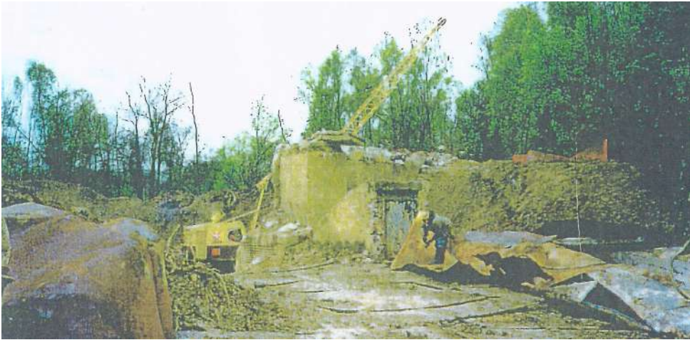
View of storage fuel tank with steel removed and concrete being destroyed
