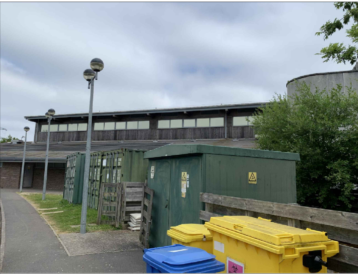
Image to proposed location, adjacent to plant room and Sub Station
