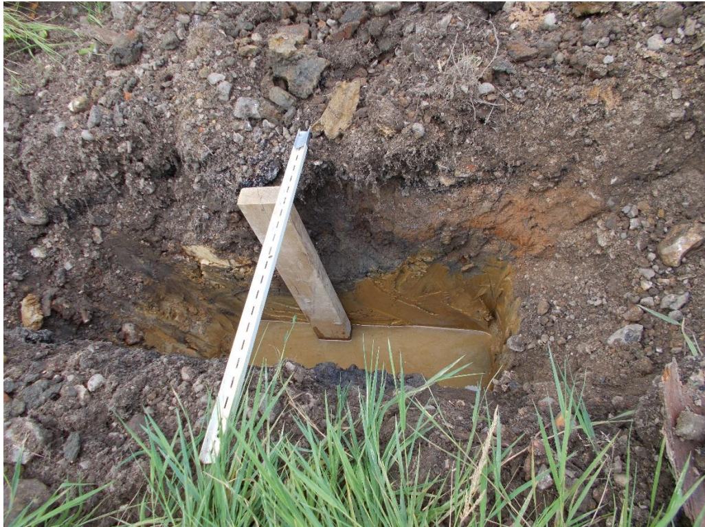
Photo 5: Percolation Test Pit PTP 1.
