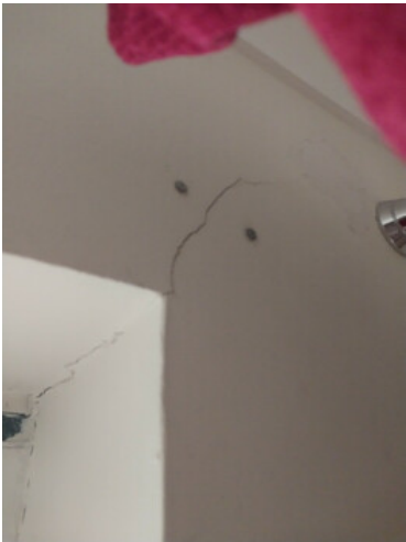
INT - Rear elevation in rear lounge - Visit #5
