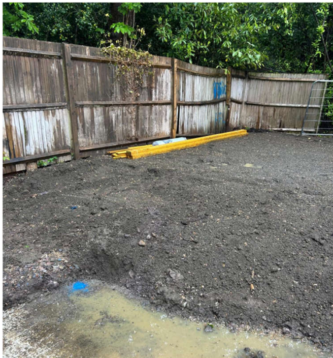
Reduced level excavation
