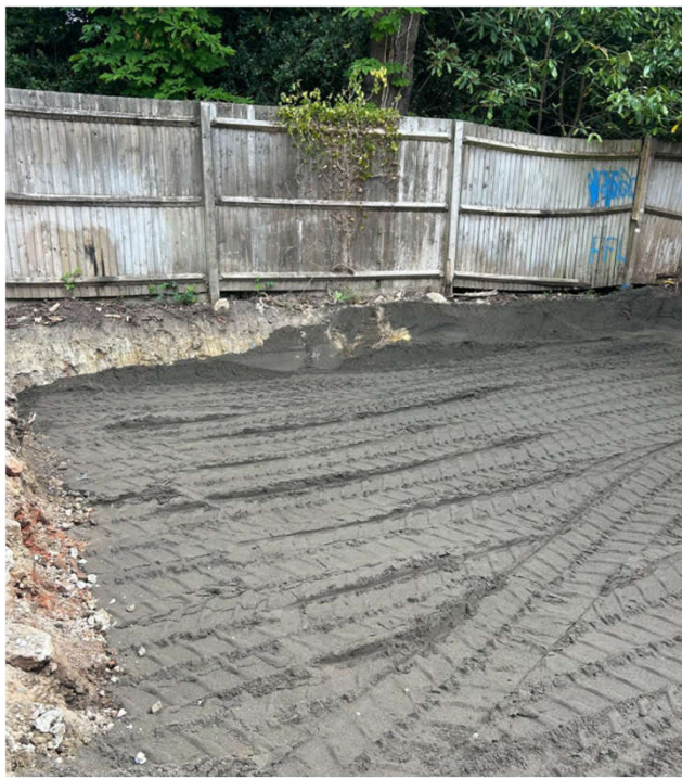
Placement of imported reject sand
