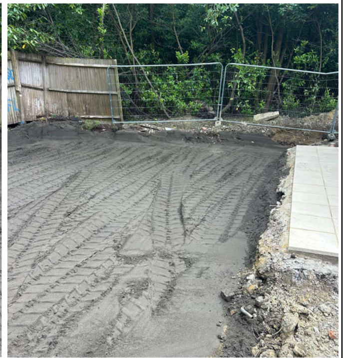
Placement of imported reject sand
