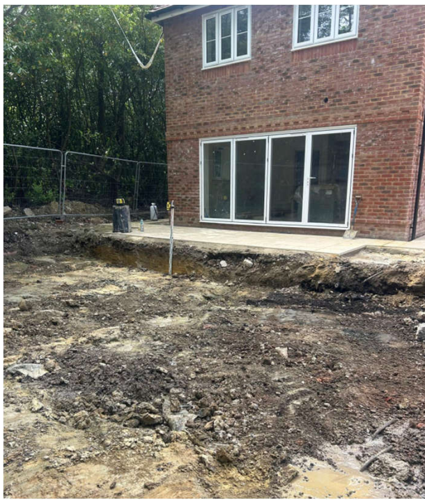
Reduced level excavation
