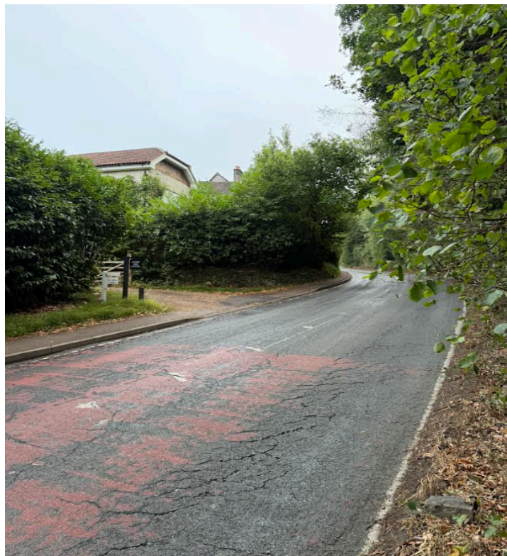
Figure 2: Site Street View
