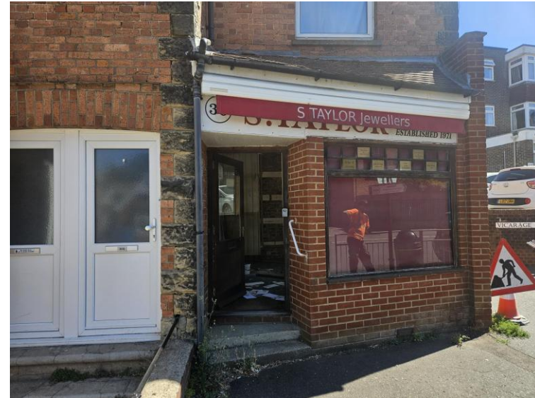
Figure 1: View of the existing site front elevation.
