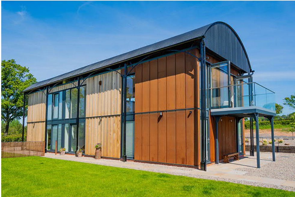
An example of a new dwelling structure within existing frame of a Dutch style barn with original columns and trussing exposed
