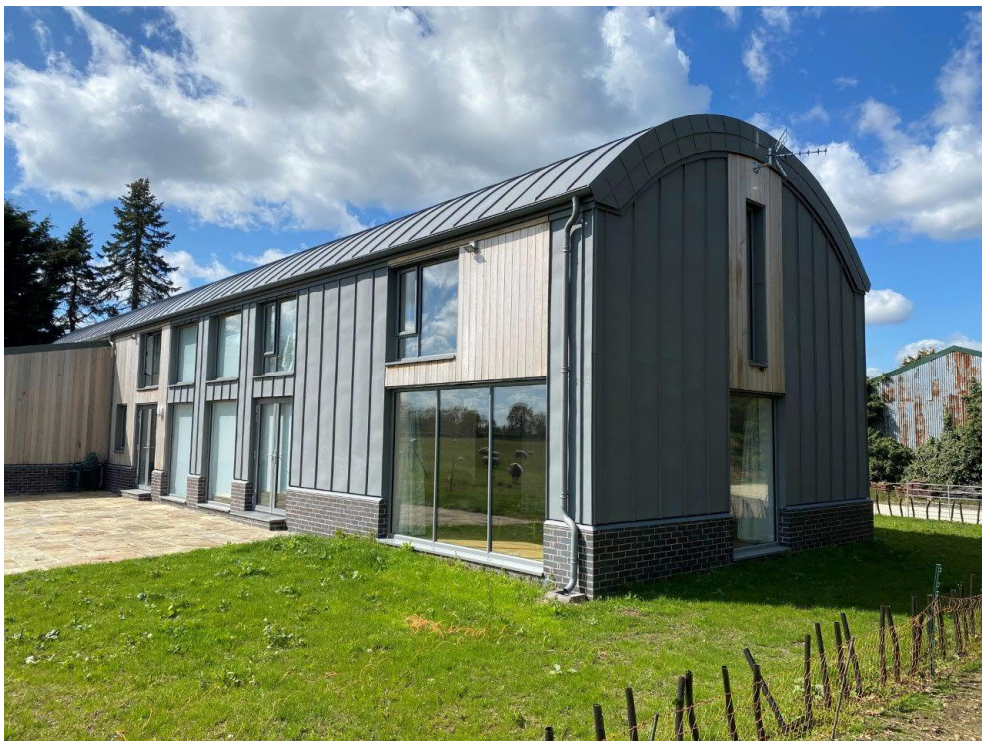
An example of Zinc or similar standing seam roof cladding, barge boards and rainwater goods
