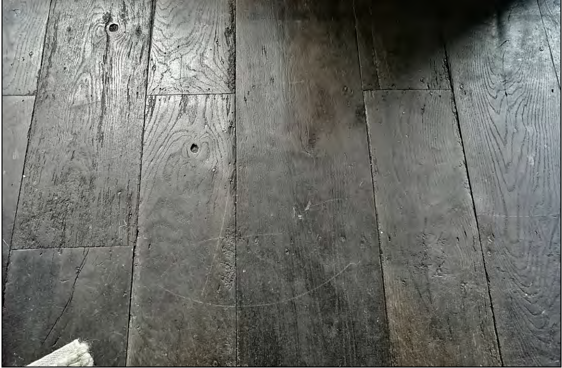
Plate 45: The floor laid c.1939 at the south end of the current dining room (bays 4 and 5), butt-jointed with no gaps, a variety of board sized and differential wear patterns inconsistent with the current location
