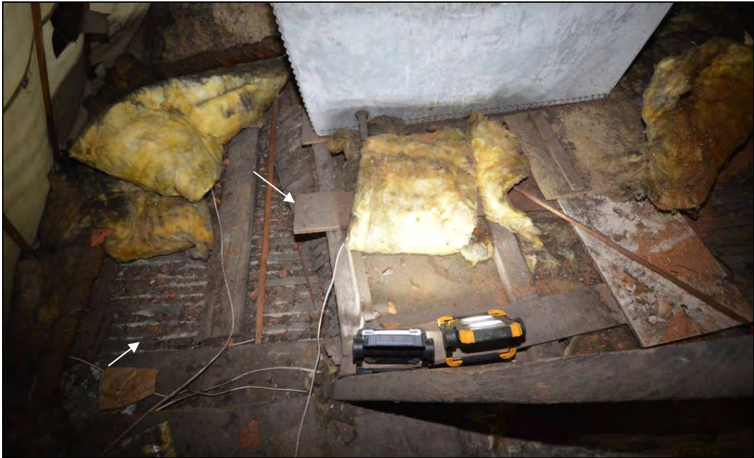
Plate 35: The two different ceiling levels in bay 4 viewed from the roof space (arrows)
