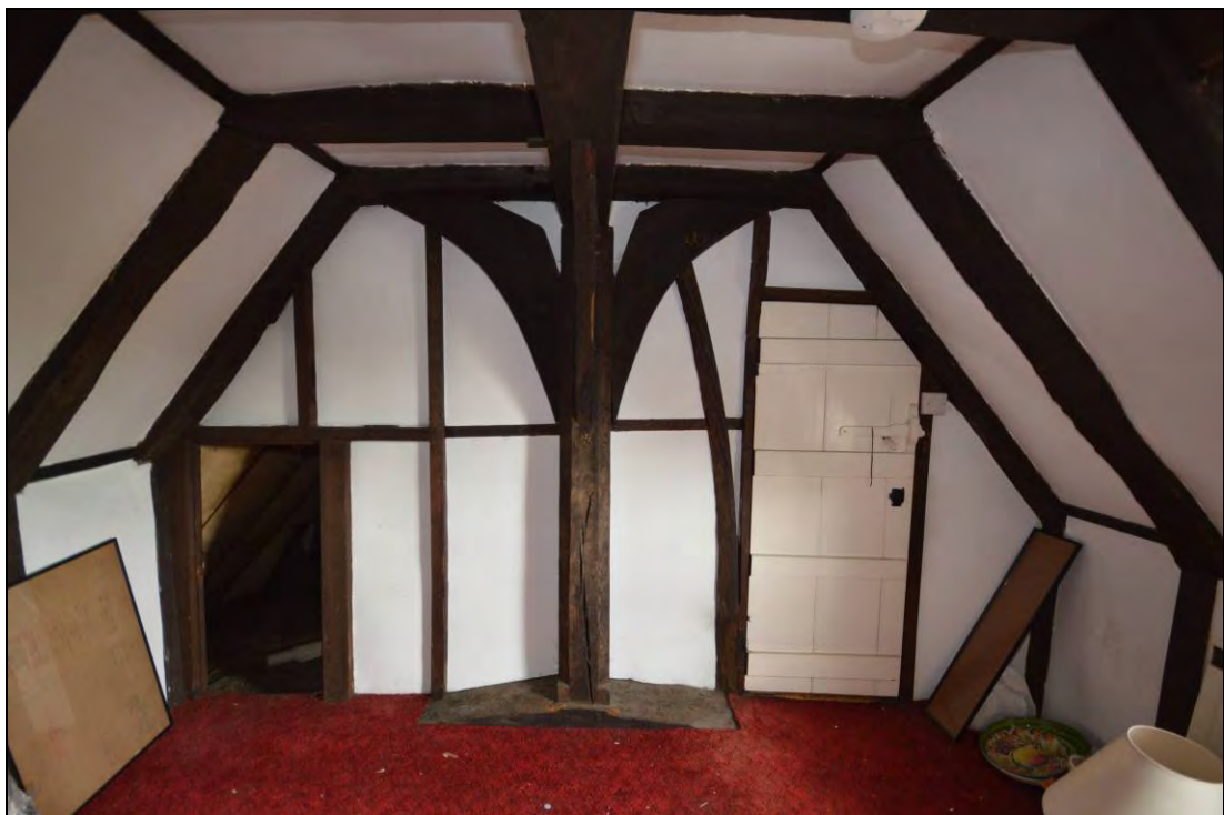
Plate 17: The former free-standing crown-post of the open-truss (T3)
