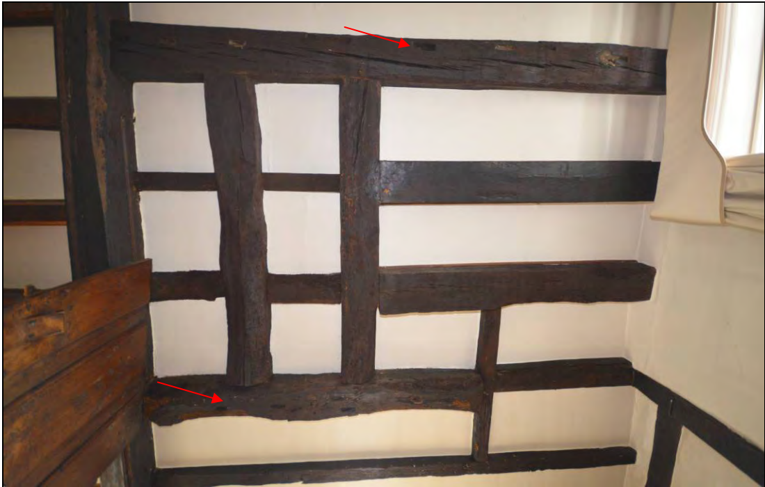
Plate 11: The stair trap and the soffit jointing to each side of it
