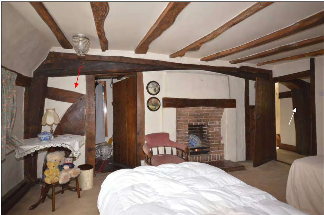
Plate 14: The south side of the open truss with the surviving parts of the head-brace and spur (red arrow); their counterparts to the east had been removed (white arrow)
