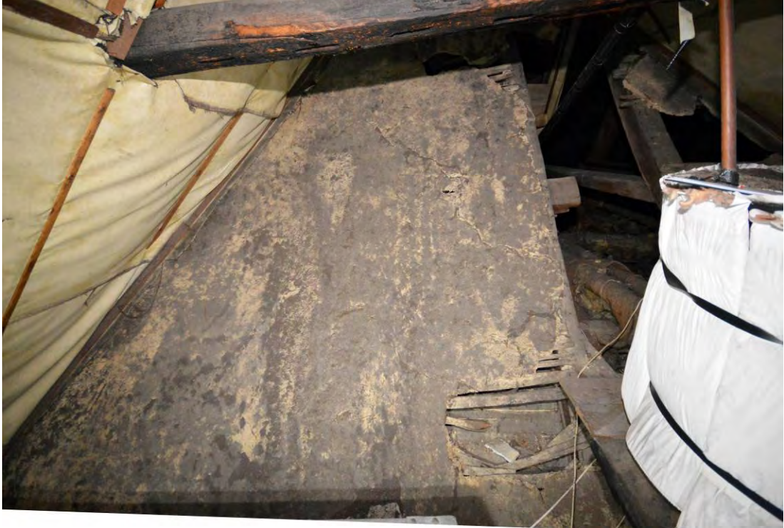
Plate 29: The lath and daub partition on the south slope of the cross-wing roof in bay 5
