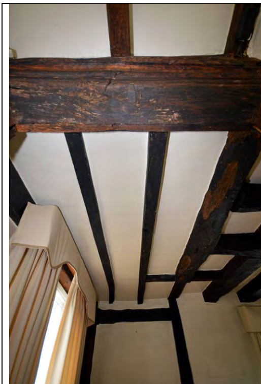
Plate 32: The eastern side of bay 1, looking south showing the two joists added to reinstate the ceiling over a probable staircase location. Note also the head-plate for a doorway in the south elevation
