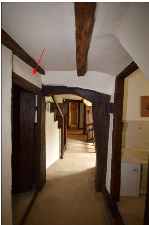
Plate 51: The entrance to the hall chamber in the partition in bay 2 (arrow)
