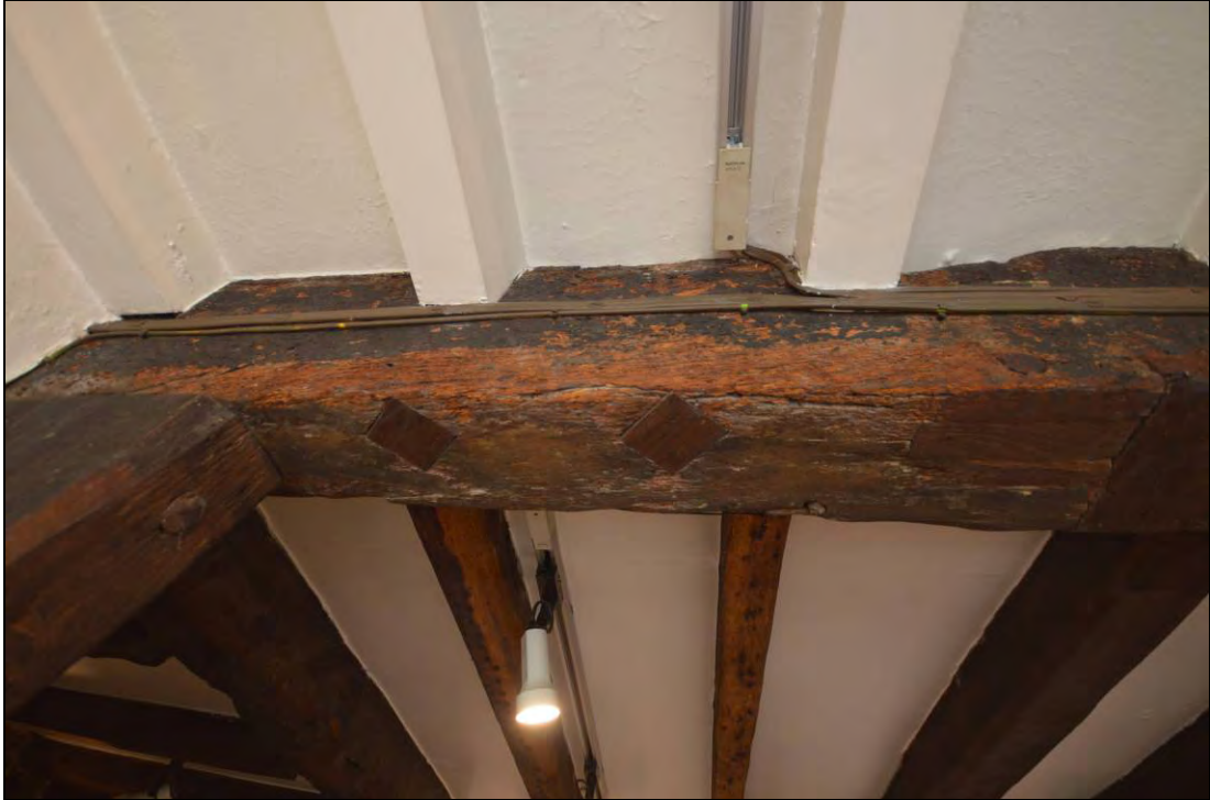
Plate 23: The soffit of the cross-beam of the T7 truss at the eastern end of the cross-wing with evidence of a three-light close-mullioned window
