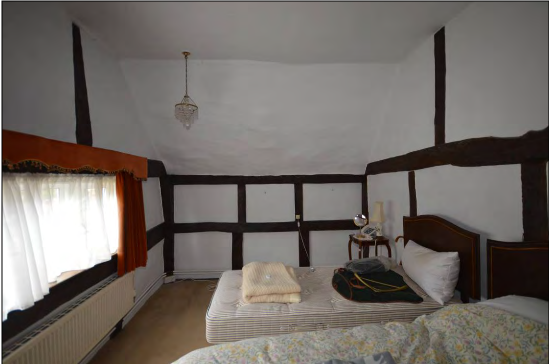
Plate 22: The small-panel framing in the cross-wing at first floor level, north end (bay 5)
