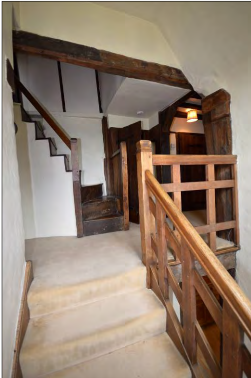
Plate 50: View towards the plasterboard ceiling adjacent to the attic staircase on the first floor
