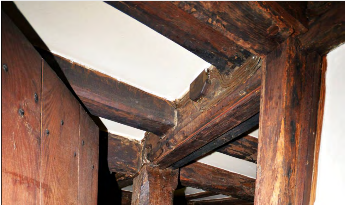
Plate 26: Detail of the cross-wing joists supporting the first floor in bay 7
