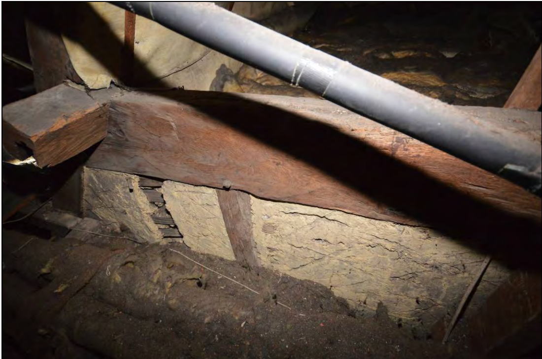
Plate 21: Lath and daub on the T6 partition truss surviving to collar level within the roof of the cross-wing
