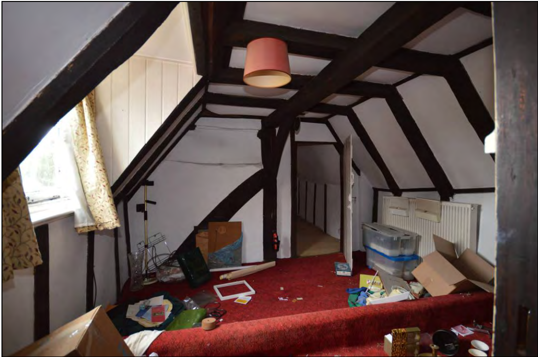
Plate 18: The north side of the T2 partition truss, the western foot-brace removed to create a doorway
