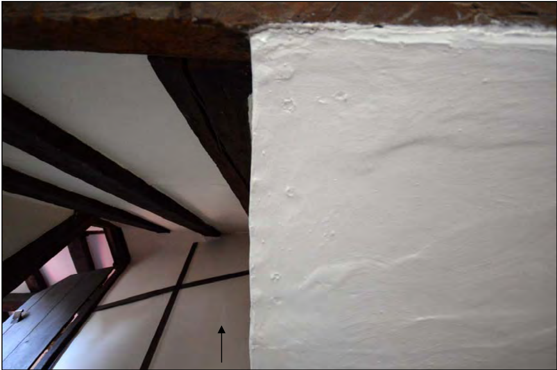
Plate 53: View up towards the attic doorway from the first floor landing showing existing modern partitions (arrow)
