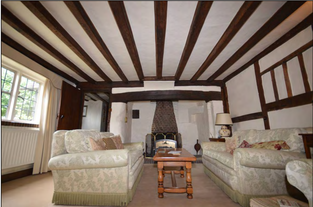
Plate 19: The new joists inserted into the open hall to create a chamber above and the masonry base of the southern hearth of the new multi-flue chimney stack
