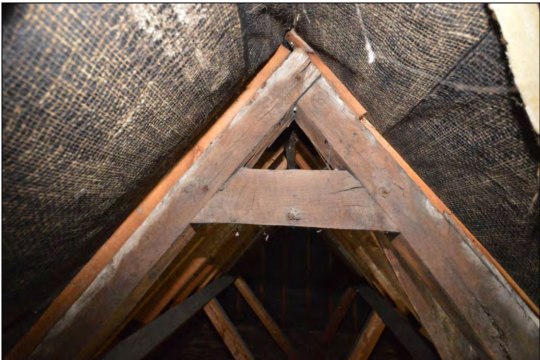
Plate 28: The high-set collar and jointing evidence for a central jack rafter indicative of a hipped roof terminal at the eastern end of the cross-wing
