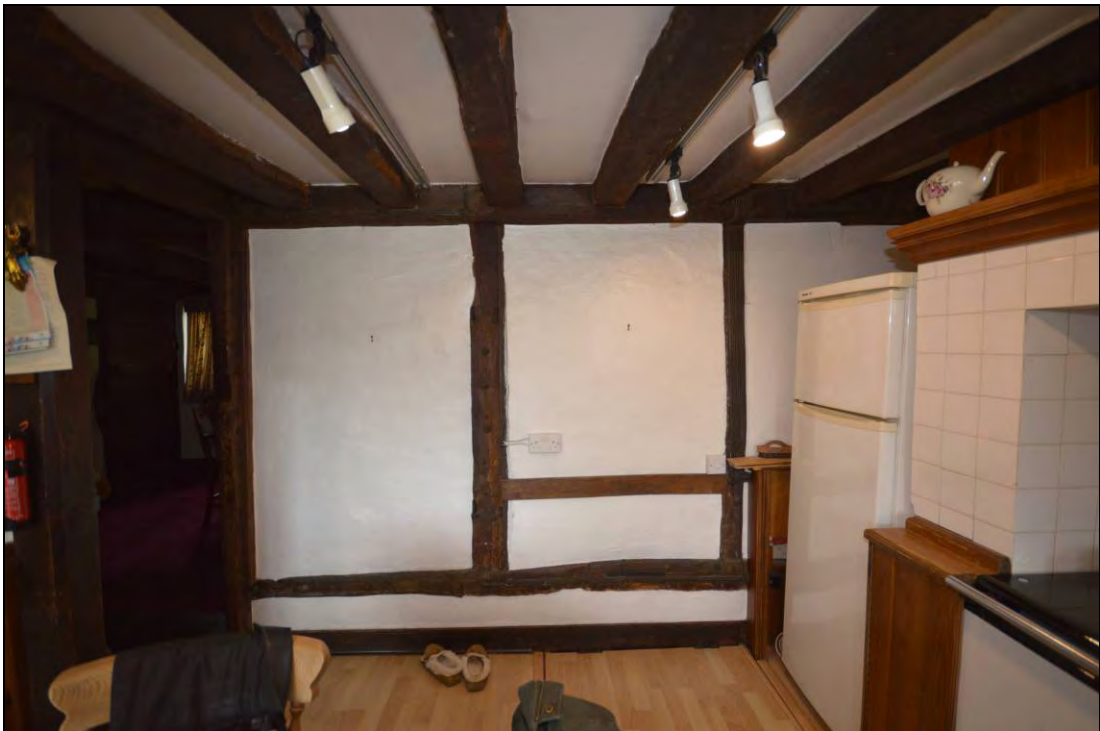
Plate 24: The two doorways in the T6 partition truss, east side
