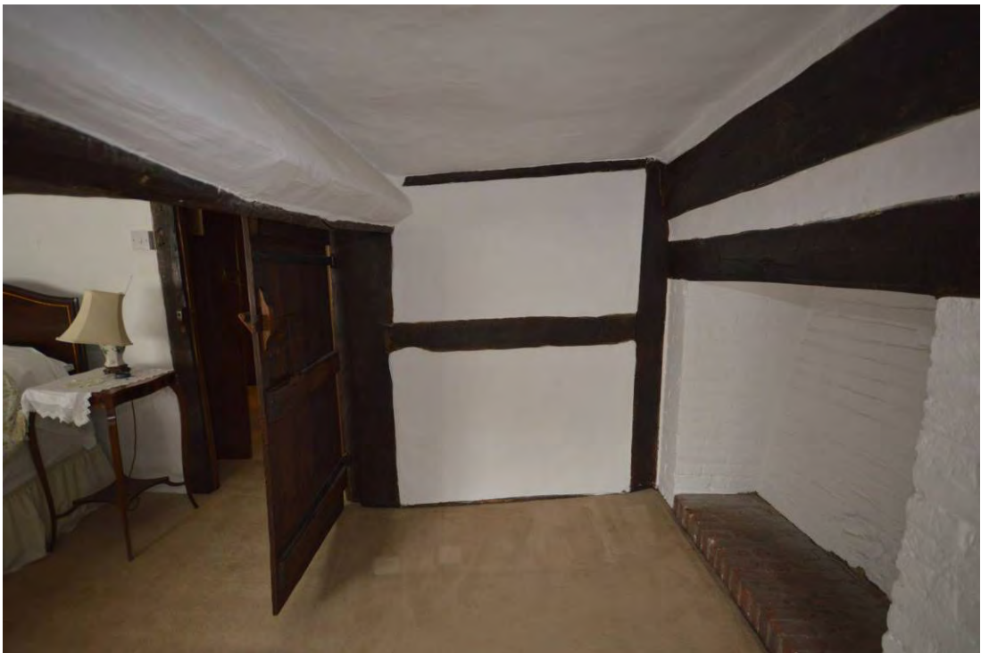
Plate 30: The lath and daub finish to the south slope of the bay 5 cross-wing roof, first floor
