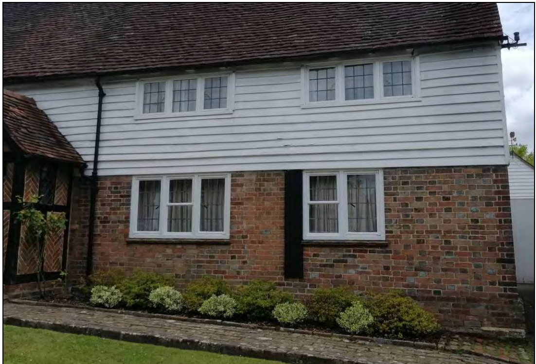
Plate 37: The front elevation showing the consistency of the brickwork across bays 1 and 2 and the differences in fenestration to those proposed in 1939
