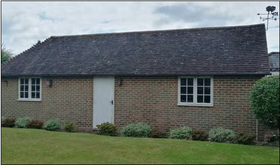
Plate 43: The north elevation of the garage
