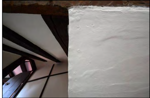
detail of the plaster-board nailed in place
