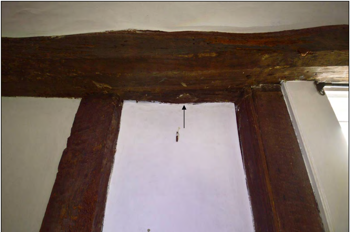
Plate 16: Detail of the wall plate soffit on the east side of bay 1 showing the diamond mortise for a window mullion (arrow)
