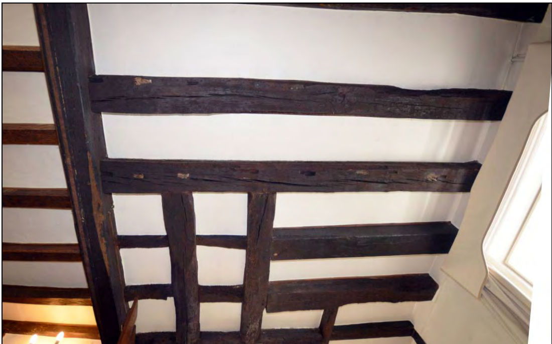
Plate 12: Two adjacent sets of mortises for partitioning on the bay 1 joists
