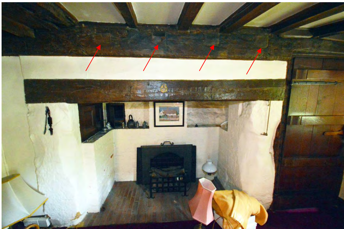
Plate 15: The north side of the T4 truss showing the original joist mortises in the cross-beam, now redundant, with new joists of lesser scantling above raising the height of the ceiling (arrows)
