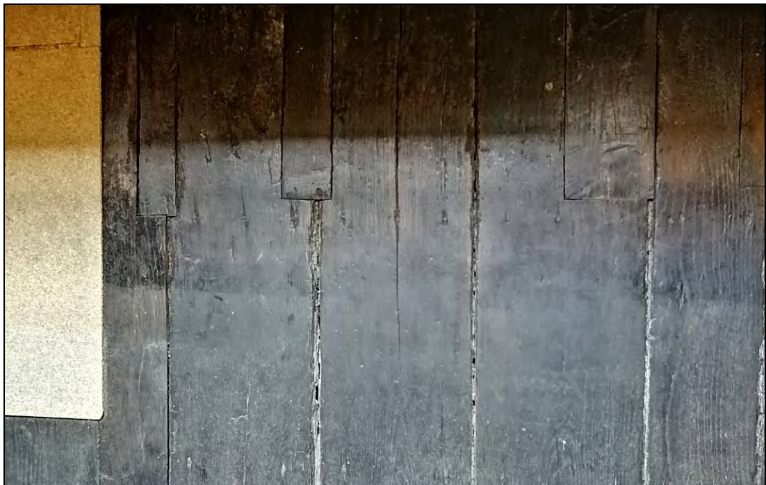
Plate 46: The floor over the cellar at the north end of bay 5, complete with consistent board sizes, wear patterns and gaps between the boards
