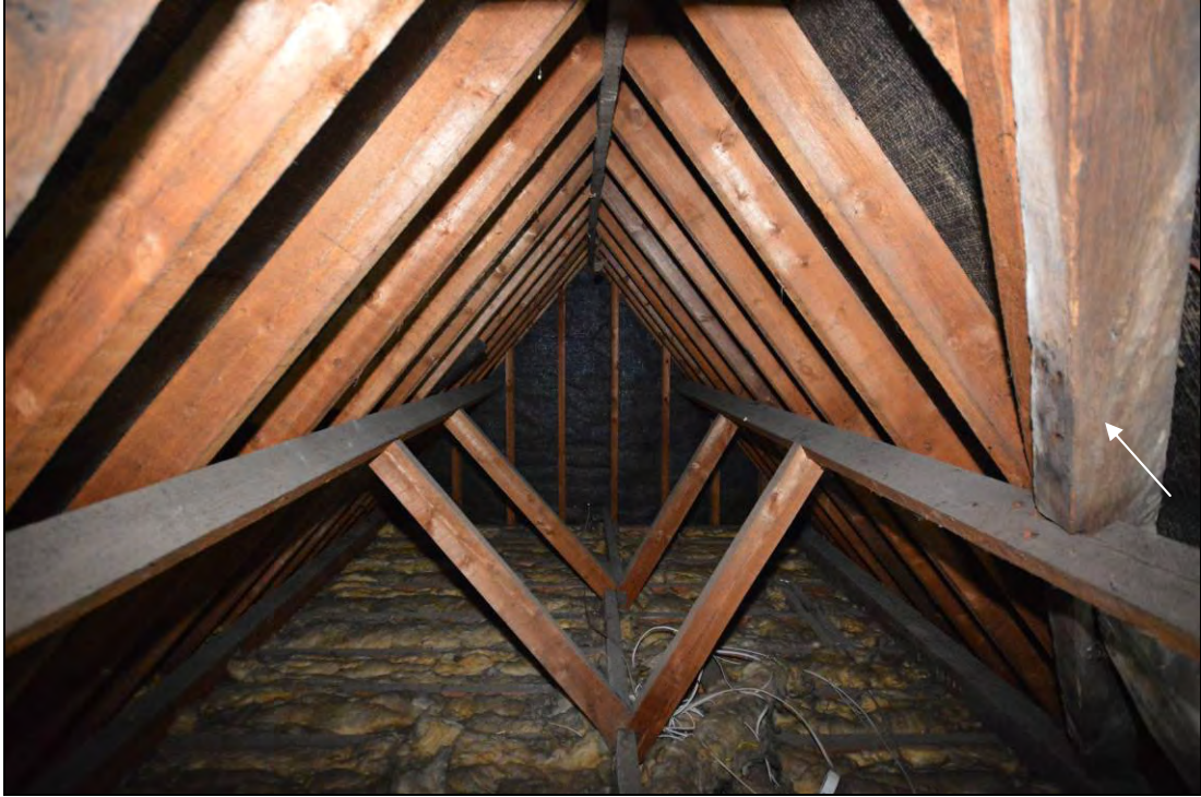
Plate 49: The interior of the roof added in 1939 over bay 6 of the cross-wing (south hip rafter of the phase 3 roof just visible – arrow)
