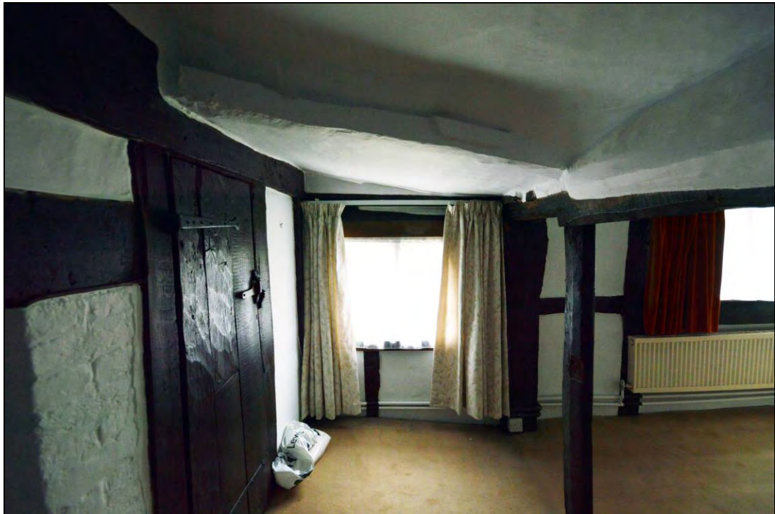
Plate 34: The stepped ceiling finish within bay 4 on the first floor of the main range
