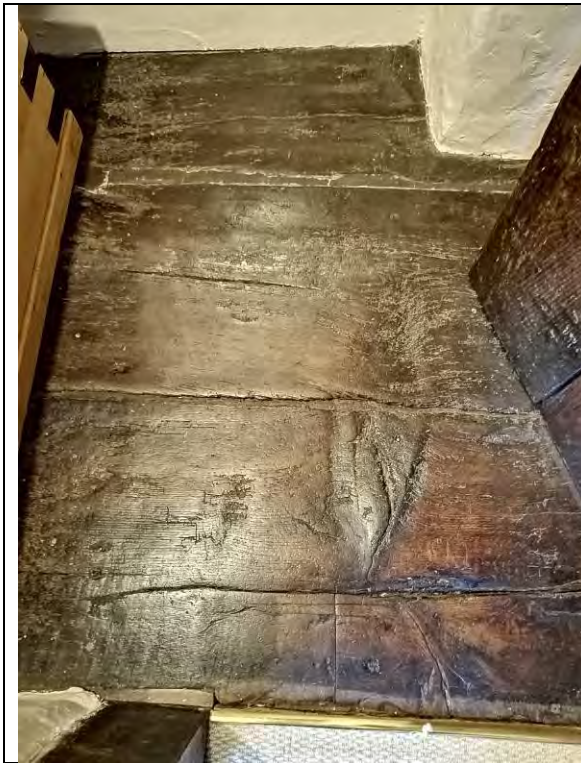
Plate 47: Detail of the in situ early floorboards within the closet at the west side of bay 3 (late 16 th century)
