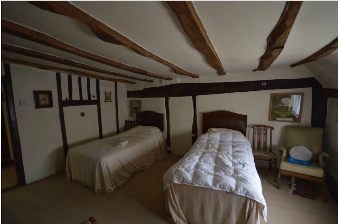
Plate 33: The attic floor joists in bay 2 looking south
