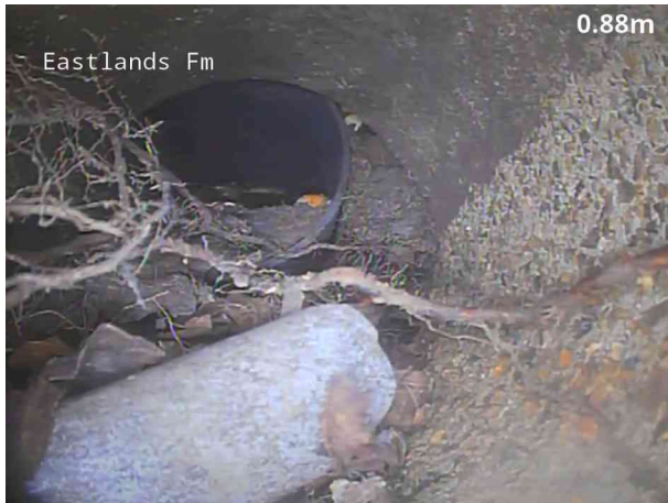
7, 00:00:46, 1.00 m Finish node, outfall, reference: Outfall 2, Buried
