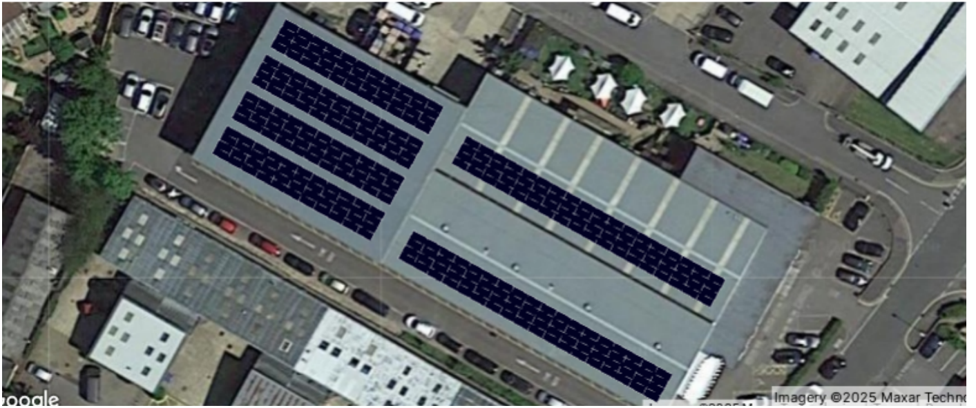
Figure 3 Location of solar panels
