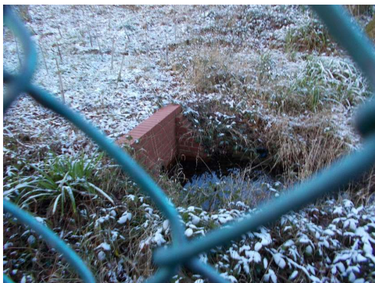
Ditch/tributary showing culvert under the footpath southeastern edge of site
