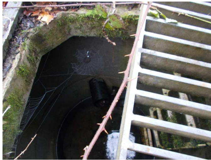
Internal view of the 4 th chamber, with drainage ditch from the Taylor Wimpey site (from the east) joining the watercourse (already draining from the south, past the Site A). The watercourse flows northwest under in embankment via this chamber.
