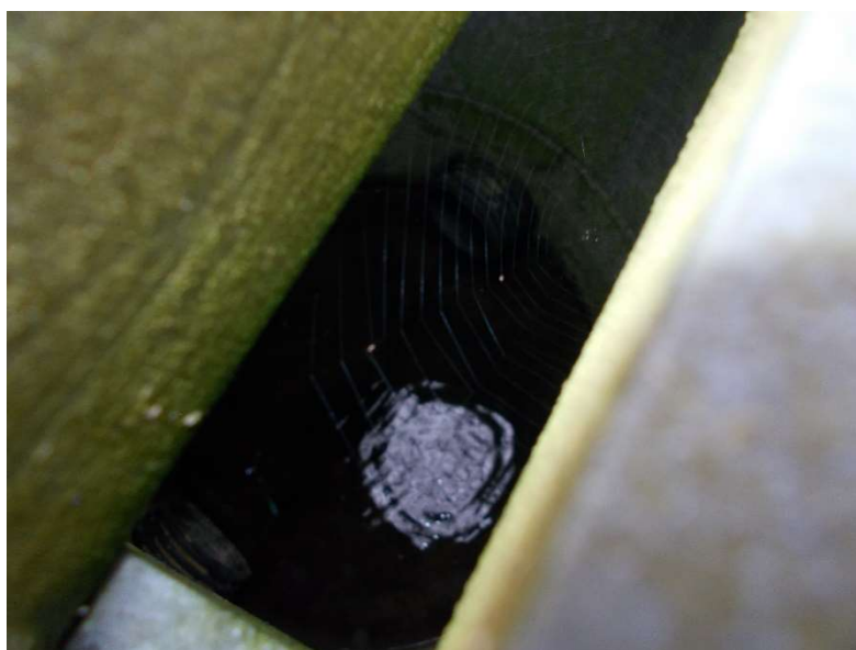
Internal view of the 3 rd chamber
