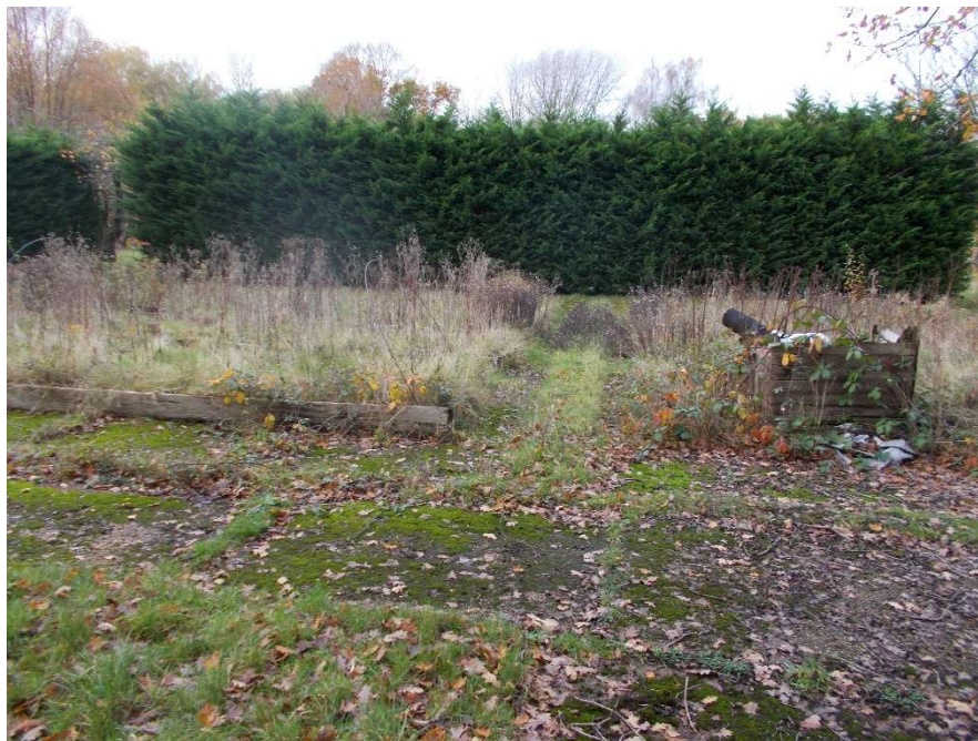
Area of hardstanding (south eastern edge of site)
