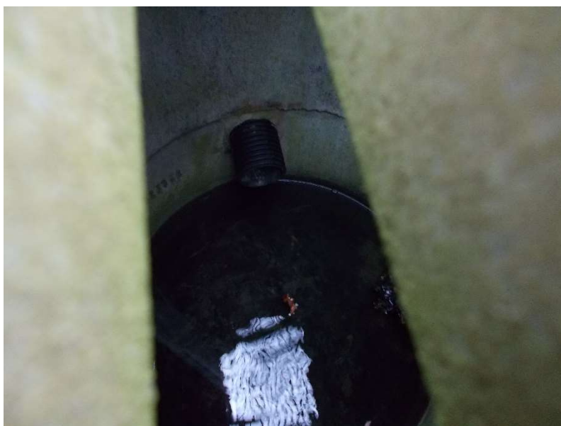
Internal view of the 2 nd chamber
