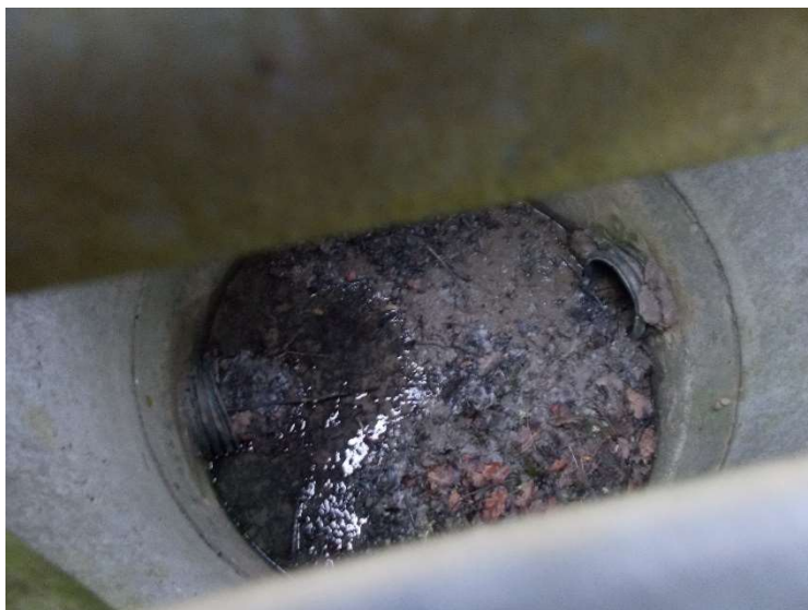
Internal view of the 1 st chamber
