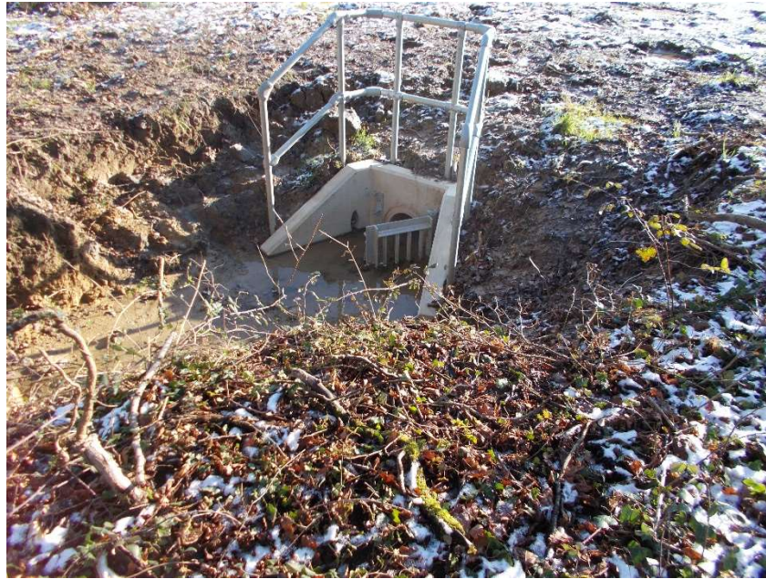
Ditch at the northeastern boundary of the site used by Taylor Wimpey for Surface water SuDS drainage.
