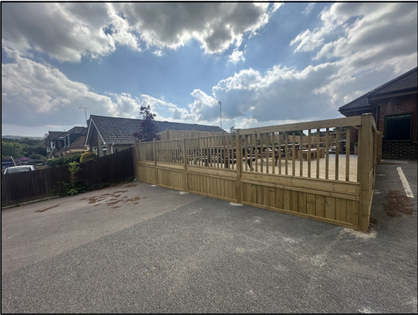
As Constructed - VIEW OF EAST DECK BALUSTRADE
