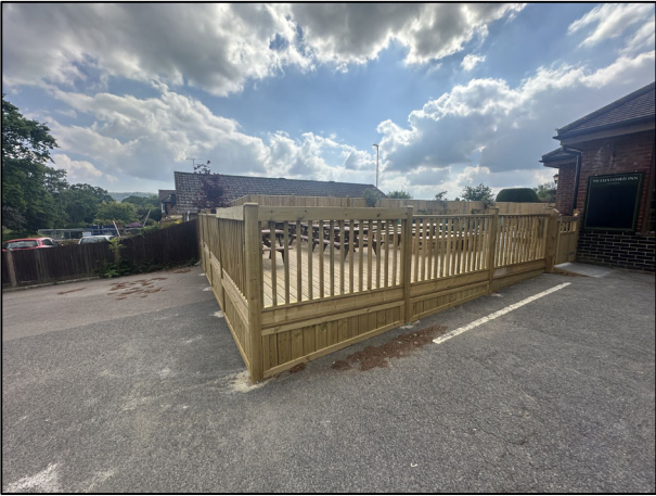
As Constructed - VIEW OF NORTH DECK BALUSTRADE
