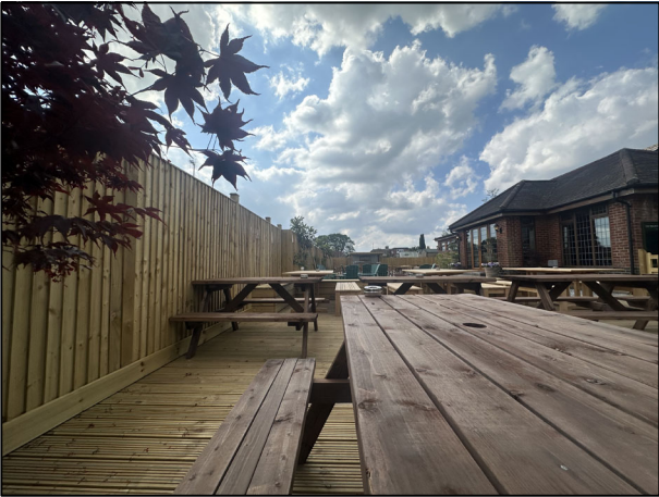
As Constructed - VIEW FROM DECK LOOKING WEST
