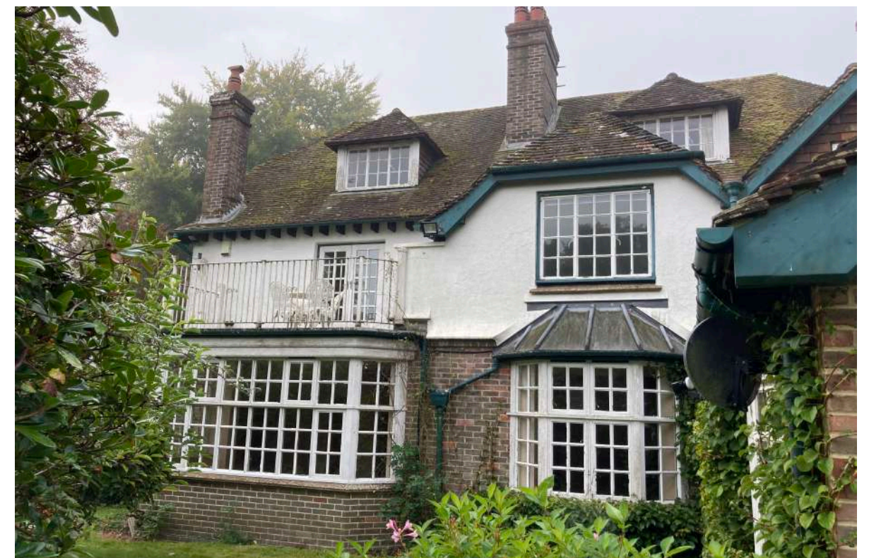
South elevation of Lane House
