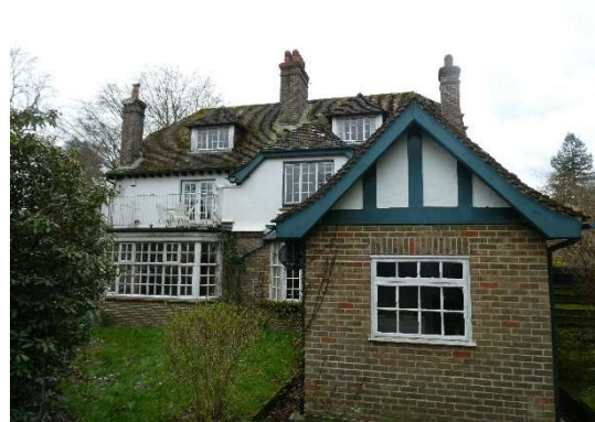
Photograph 2: North elevation of B1 showing ground-floor northern gable ended extension and main roof dormers.
