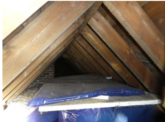
Photograph 4: Roof Void 1 at B1 showing the immediate water tanks and reduced size of the roof void.
