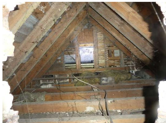
Photograph 6: Southern extent of Roof Void 2 at B1.
