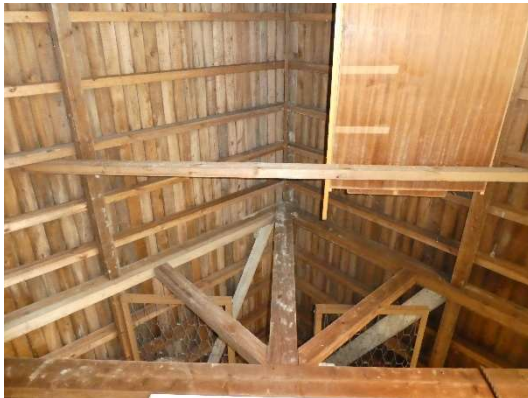
Photograph 9: Roof area within the northern garage space.
