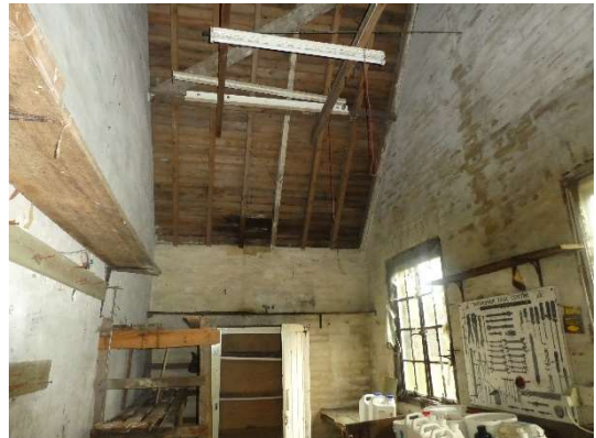
Photograph 10: Storeroom within the southern extent of B2.
