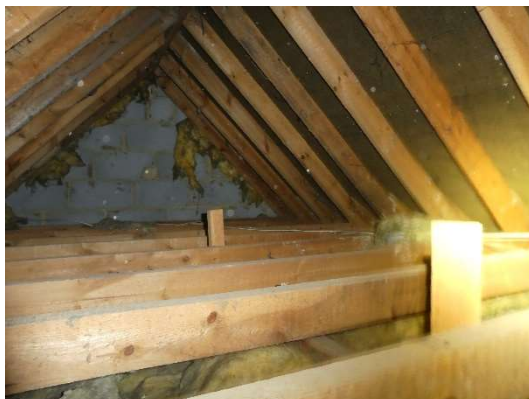
Photograph 5: Northern extent of Roof Void 2 at B1.
