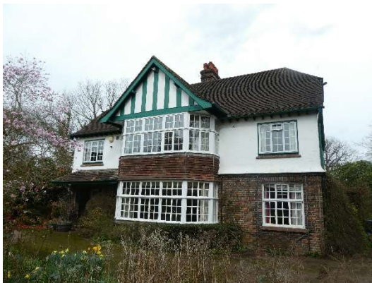
Photograph 1: South elevation of B1, showing tile hanging between the bay windows.
